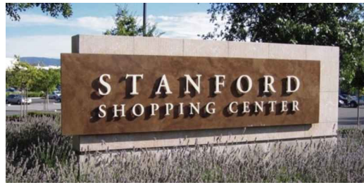
APPLIED LETTERS EXAMPLE: LASER CUT STEEL LETTERS APPLIED W/ 3/4-1" STANDOFFS FROM CORTEN PLATE, PAINTED WHITE
