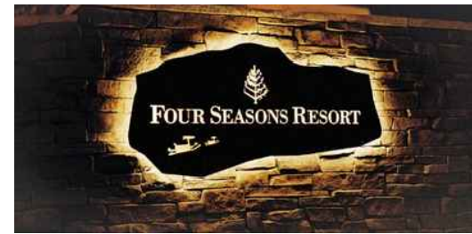
BACKLIT SIGN PANEL EXAMPLE: APPLIED LETTERS TO BE ADDED 3/4-1" ABOVE CUT LETTERS. LED LIGHTING TO SPILL FROM BEHIND SIGN PANEL AND CUT LETTERS
