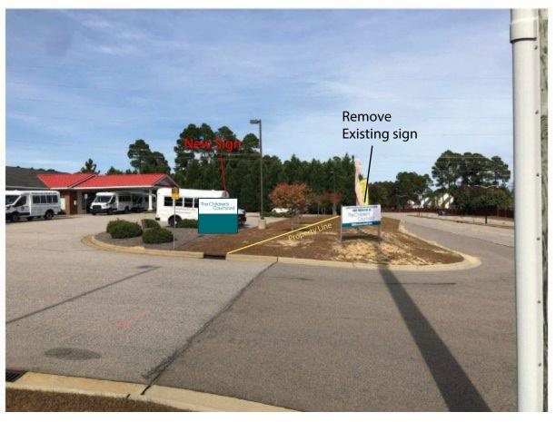
Removal of existing banner sign. Installing new illuminated cabinet sign 20 ft. from edge of pavement and 10 ft. from property line. See additional plot plan for more details.
