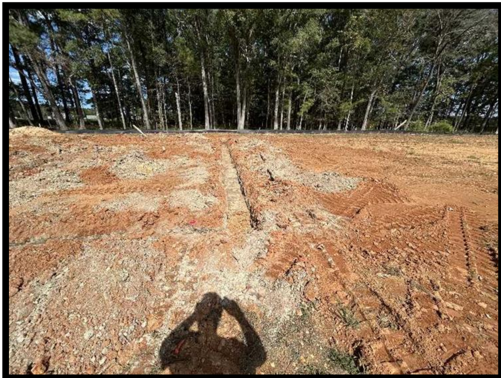
East Footings (Tests 1-2)
