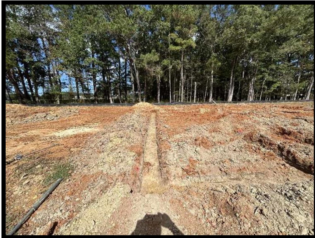
West Footings (Tests 3-4)
