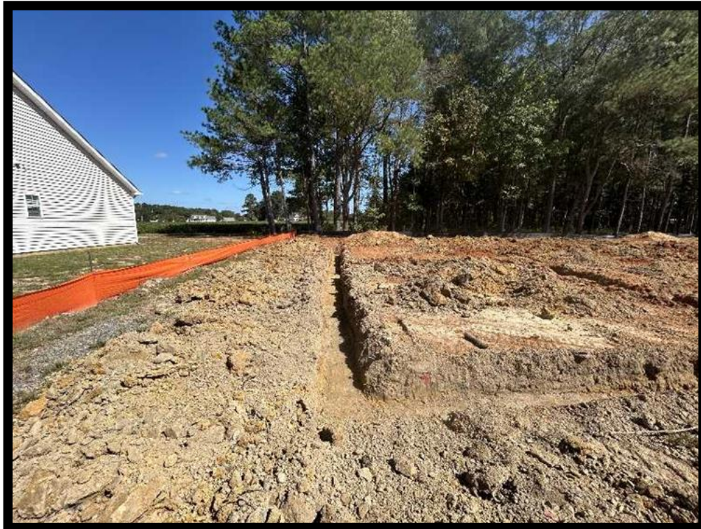
West Footing ( Test 3-4)
