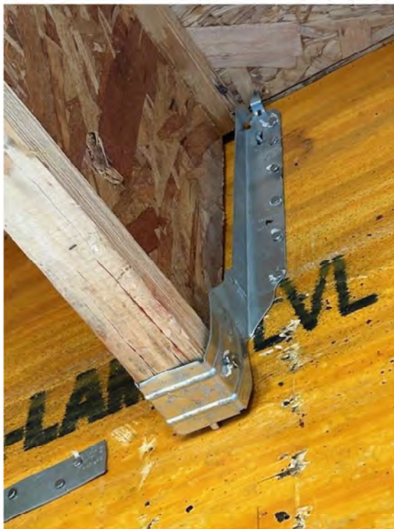
Image 4: Bottom flange nailing in 14" BCI® 4500s joists, provided by Builders FirstSource
