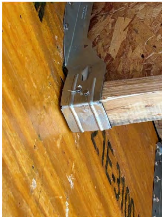
Image 2: Bottom flange nailing in 14" BCI® 4500s joists, provided by Builders FirstSource
