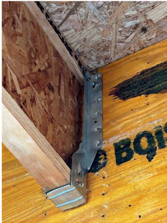
Image 3: Bottom flange nailing in 14" BCI® 4500s joists, provided by Builders FirstSource
