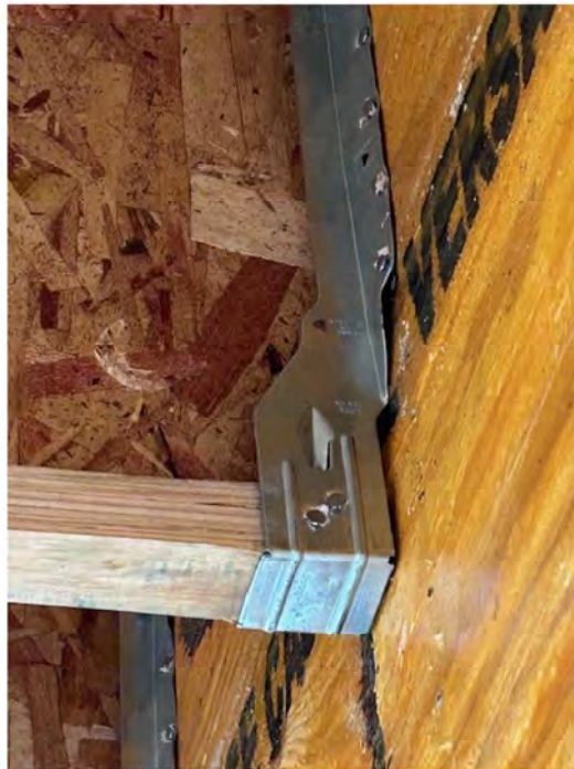
Image 1: Bottom flange nailing in 14" BCI® 4500s joists, provided by Builders FirstSource
