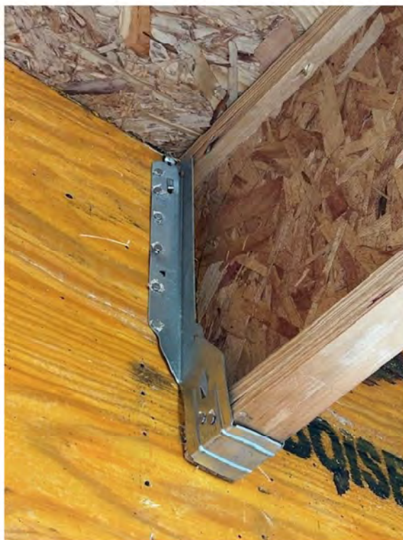
Image 6: Bottom flange nailing in 14" BCI® 4500s joists, provided by Builders FirstSource
