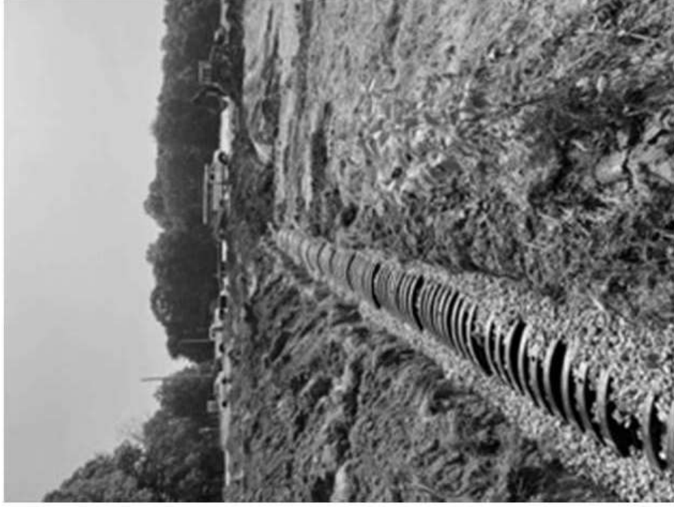
Gravel over Chamber Trench Louvers Detail:
