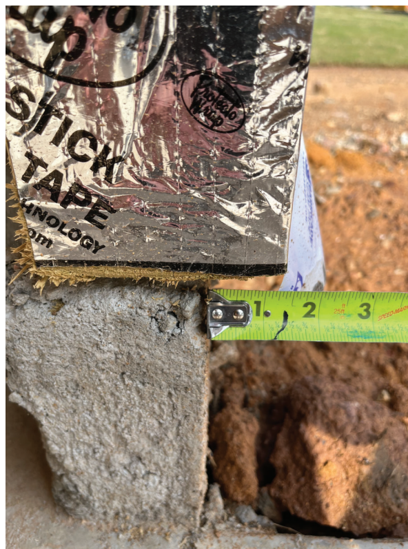
Photo 2: example of garage portal wall overhang, provided by Ryan Homes representative
