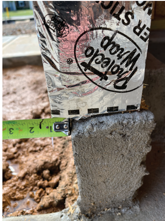
Photo 1: example of garage portal wall overhang, provided by Ryan Homes representative
