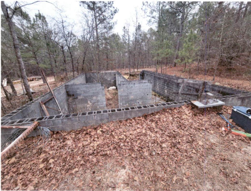
Foundation Observed (rear view)
