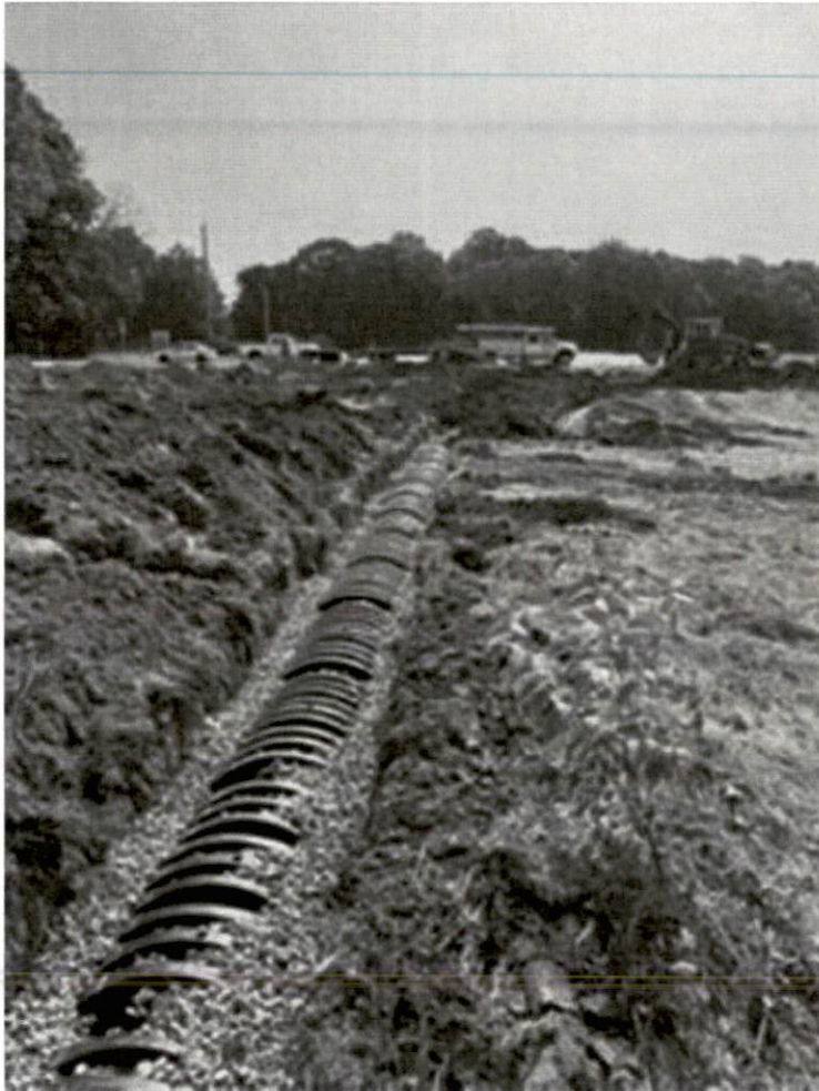
Gravel over Chamber Trench Louvers Detail:
