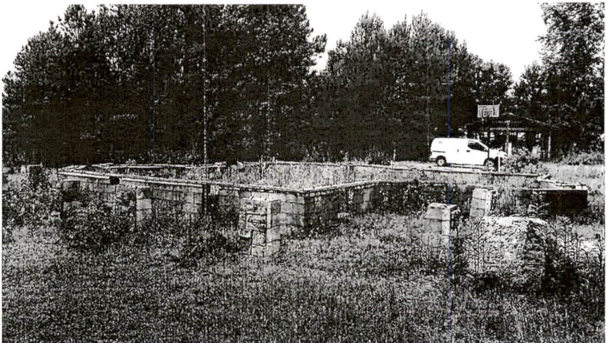
Site of Inspection
