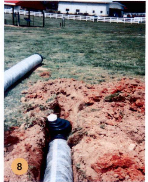
8 A Blind Tee with a screw off Clean Out Plug is placed at the end of each individual line. This allows for a line inspection.
