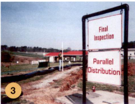
3 Laser Level check of trench depth grade and bag encased protected pipe moved onto trench site. The plastic bags protect the filter wrap from extended storage UV deterioration and natural handling abuses.
