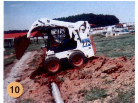
10 Narrow trenches allow for faster, less cumbersome of equipment about the site during the final cover phase, and this saves equipment time on the job.
