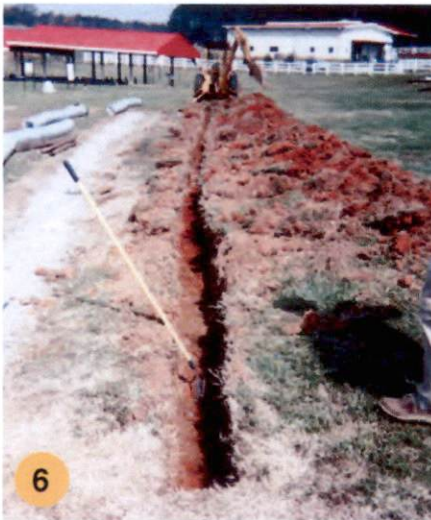
6 Trenching complete, and ready for Side-Wall rake prep sequence.
