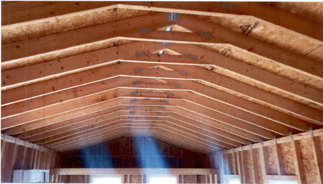
Item 2) Example of existing roof trusses
