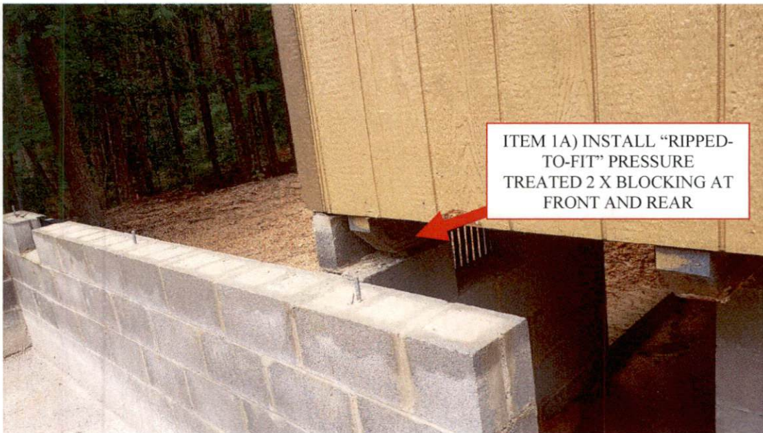
Item 1) Examples of cantilevered girders
