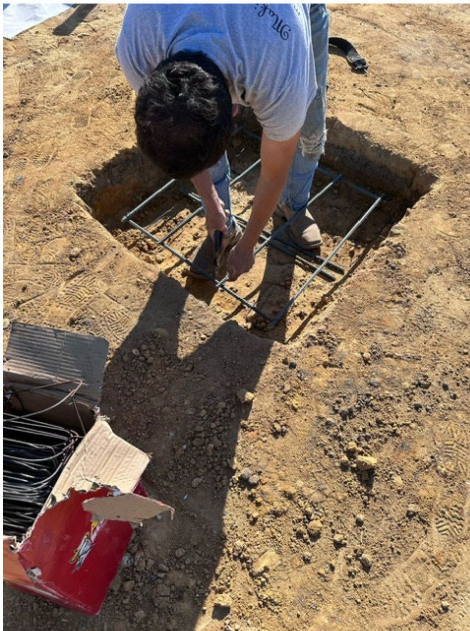
Figure 3.0 Installing footings
