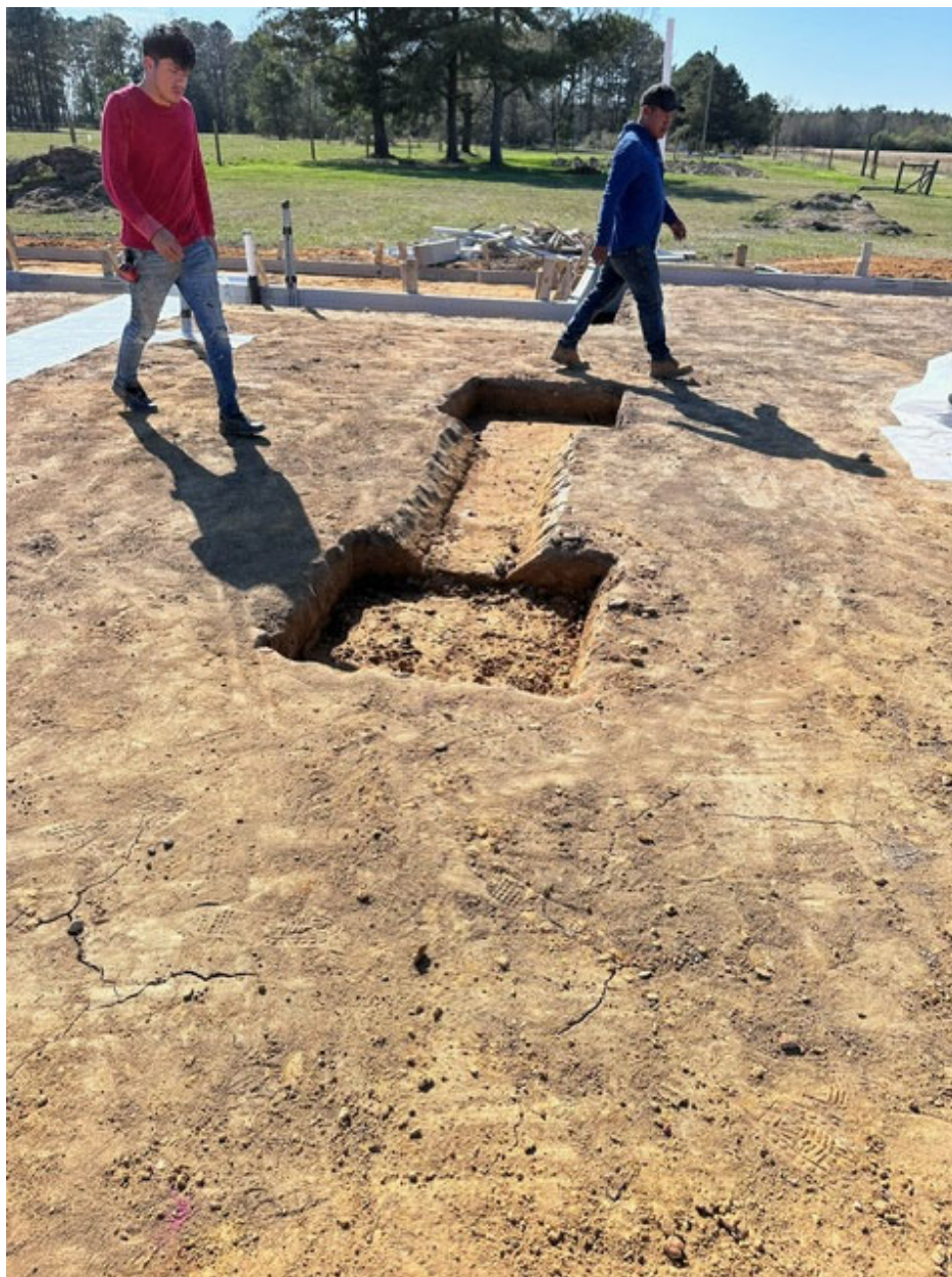
Figure 4.0 Installing interior footing.
