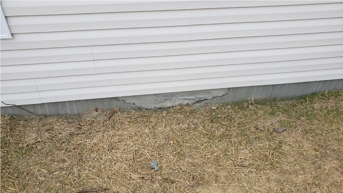
Examples of existing repairs
