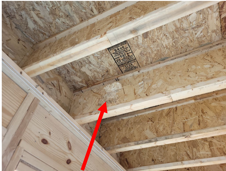
Damaged Joist
