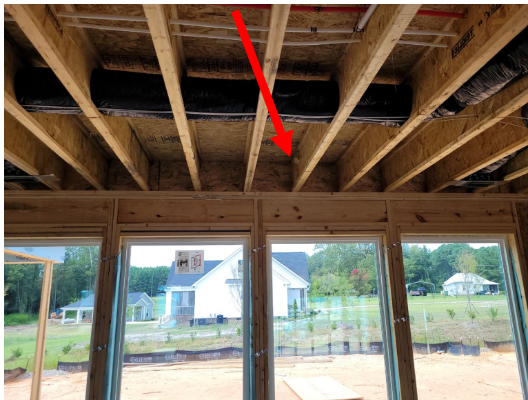
Damaged Joist
