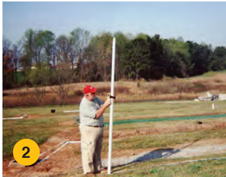
2 Laser Level adjustment setting prior to trenching sequence.
