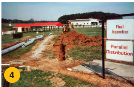
4 Protective plastic bags removed just prior to trench placement.
