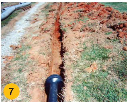
7 CPP No-Rock Septic pipes allow for narrow trenches that offer a closer OC spacing, which requires a reduced land area foot print compared to conventional 3-foot wide trenches.
