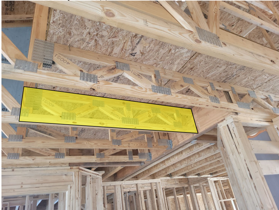
Fully sheathe (1) side of bottom “floor section” of truss
