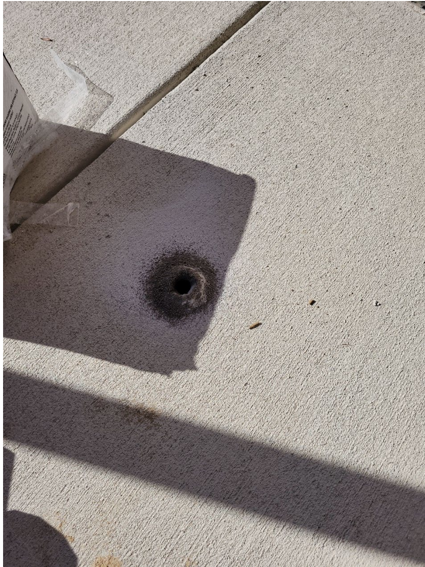
Example of area tested
