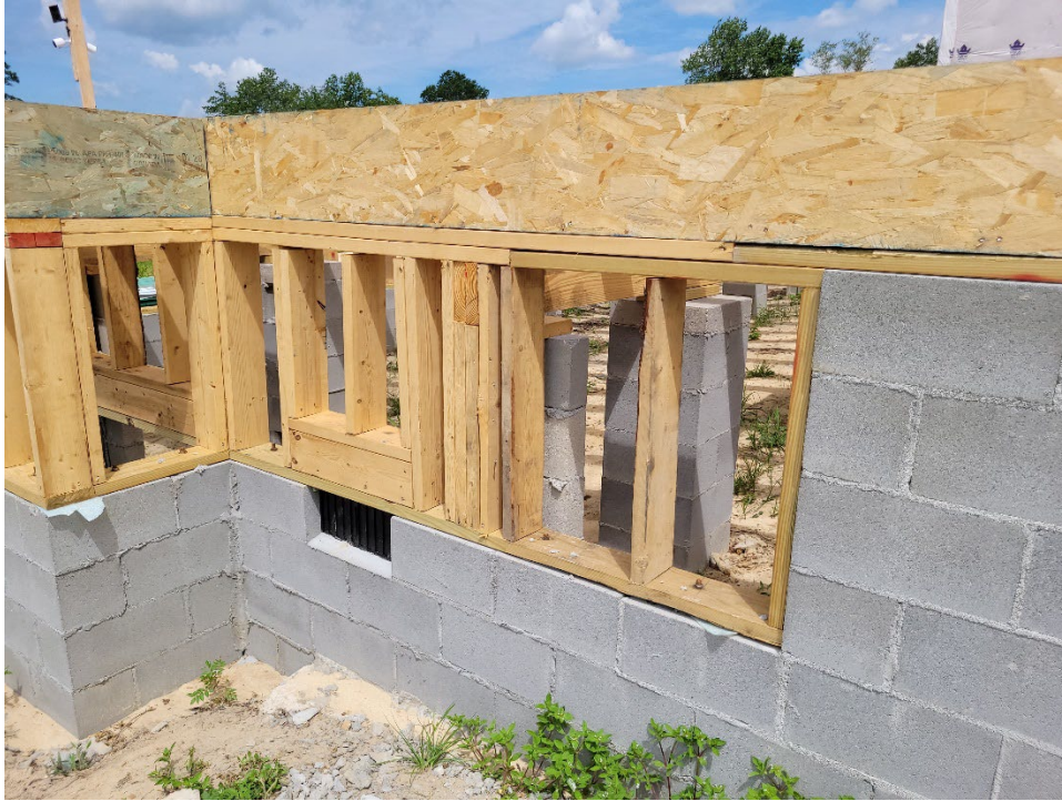
Item #6 - New plys to be added to each side of girder
