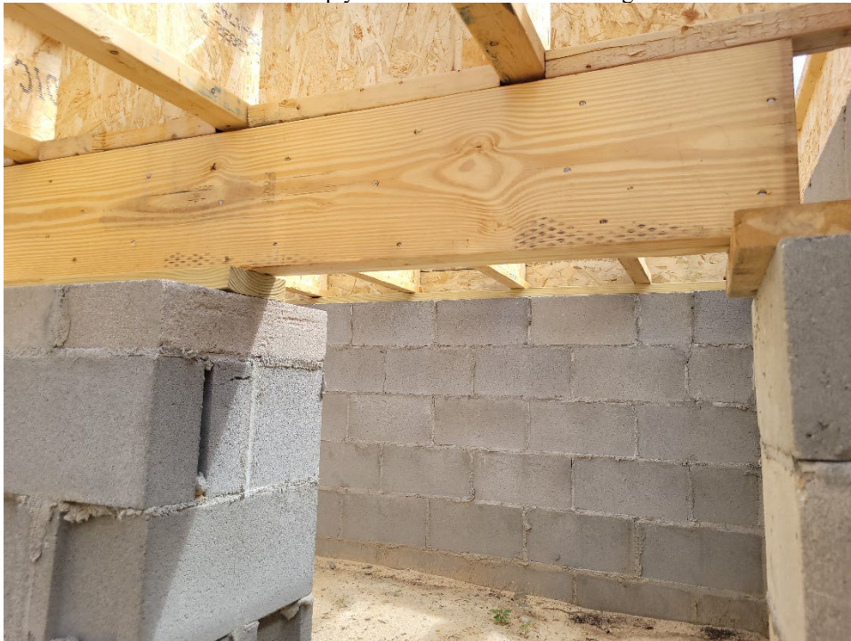
Item #6 - New plys to be added to each side of girder
