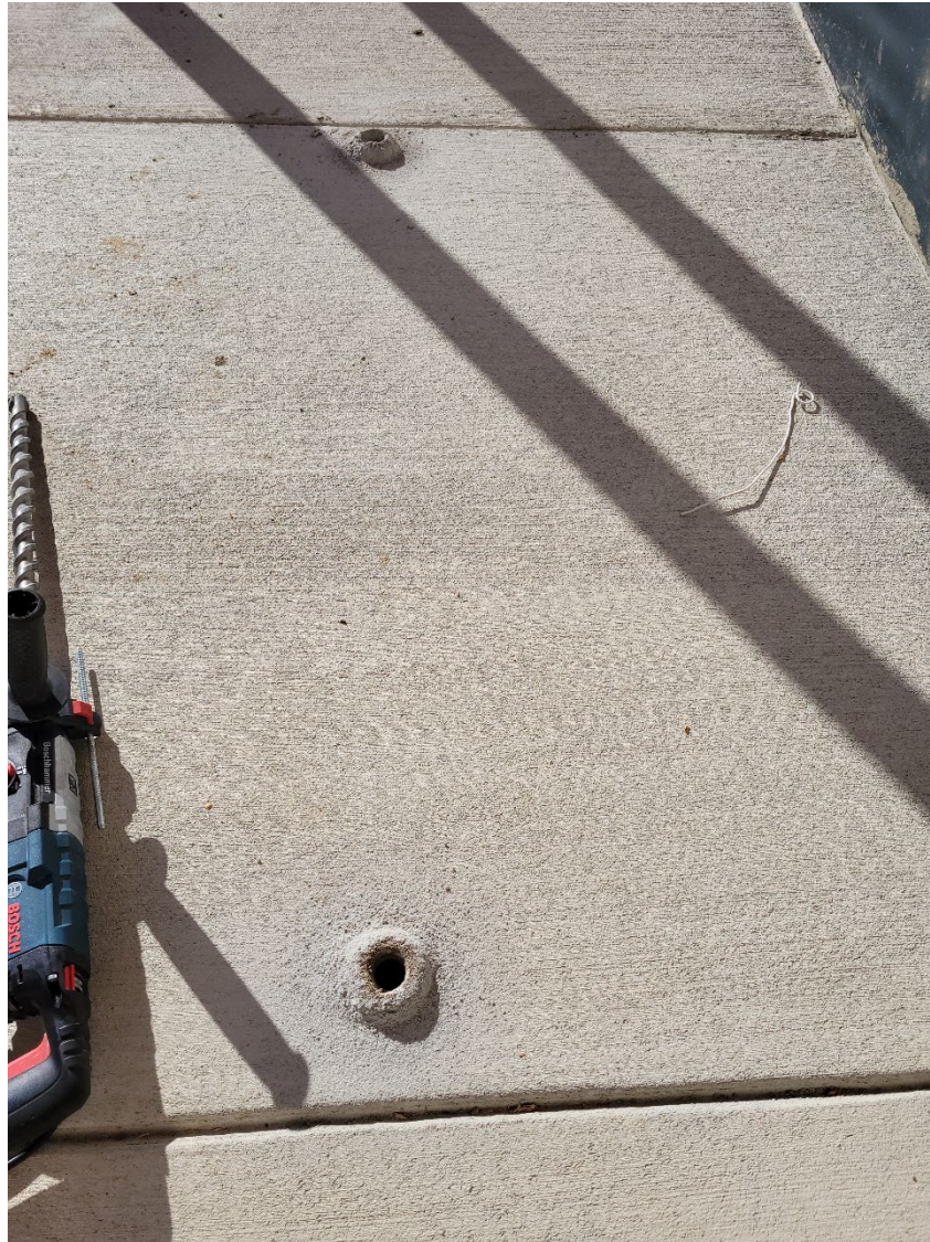
Example of area tested
