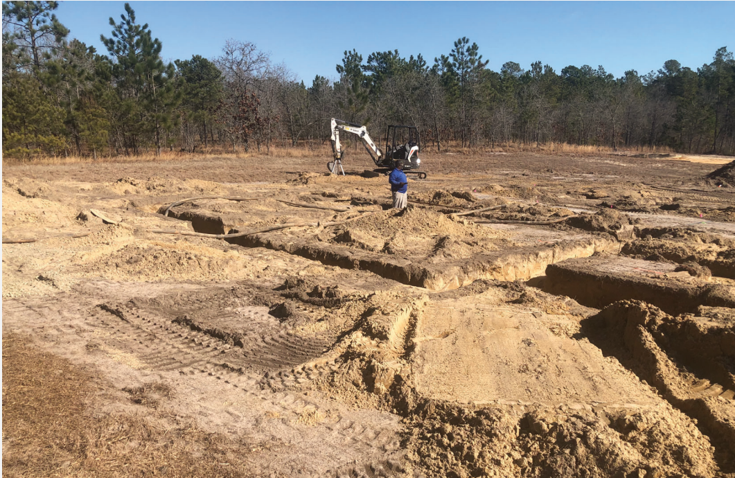
Site conditions observed
