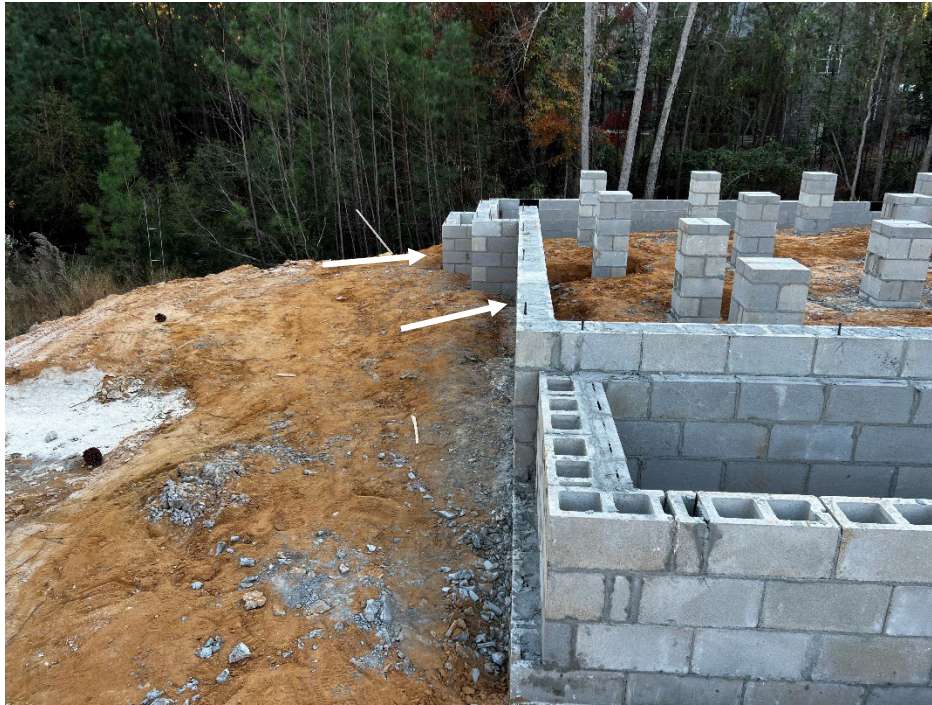
Picture 7: Trench Along Footing
