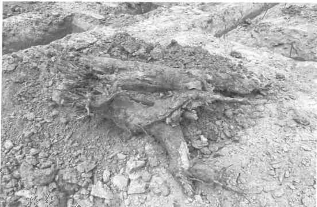
Site conditions observed on this date
