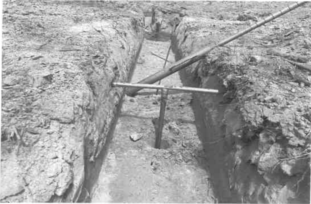
Site conditions observed on this date
