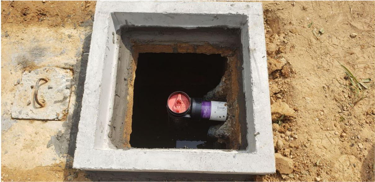
View of PVC Outlet Tee and Outlet Riser Installed
