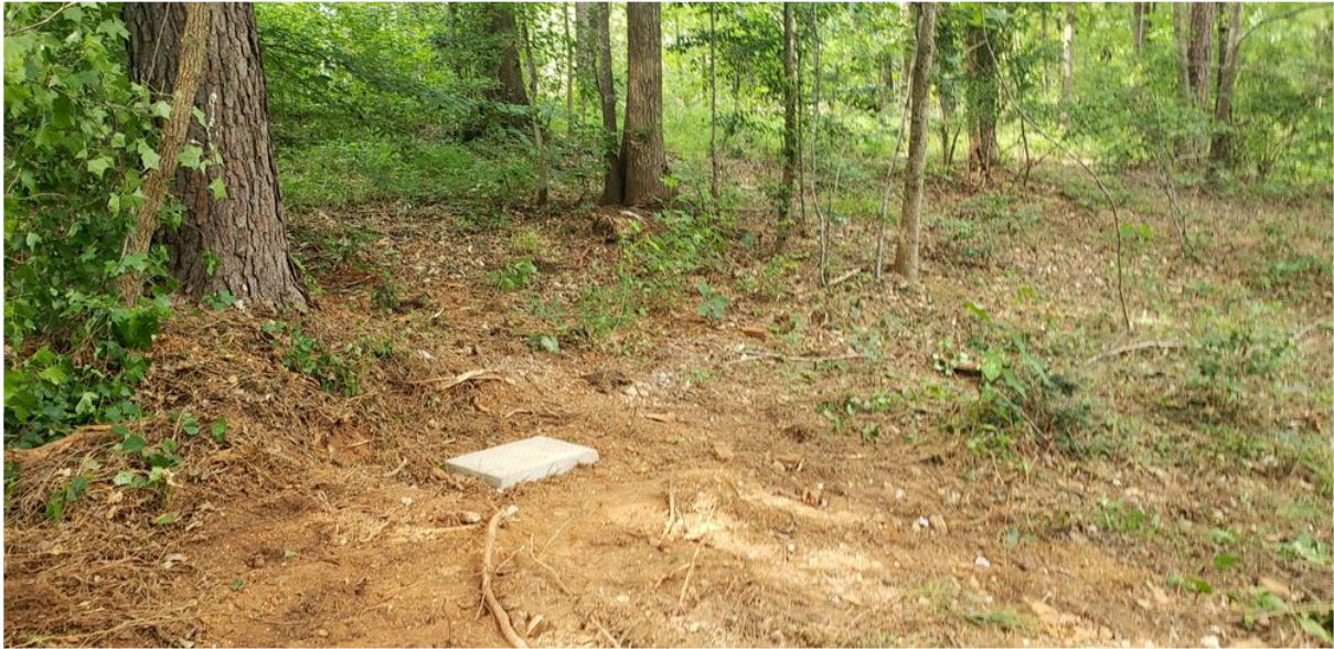
View of Location of Distribution Box
