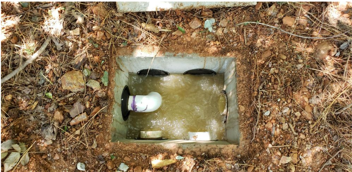
View of Restored Flow to the Dispersal Field
