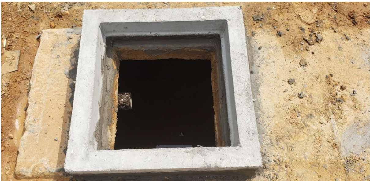
View of Inlet Riser Installed
