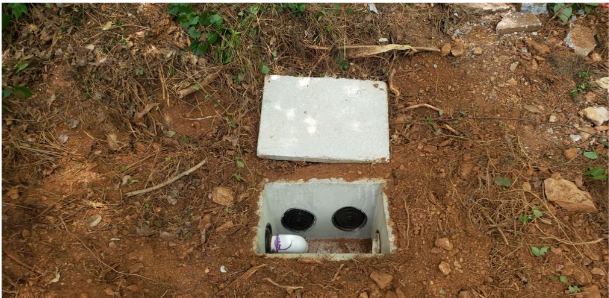
View of New Distribution Box Installed
