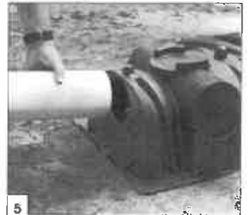
Insert inlet pipe.
