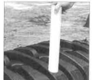
Chamber inspection port.
