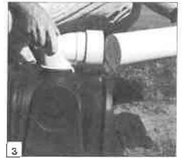
Connect inlet pipe.
