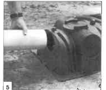
5 Insert inlet pipe.
