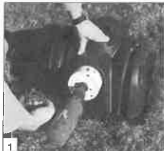
Drill endcap on side or top.
