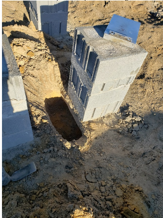
Example of Repaired Footing
