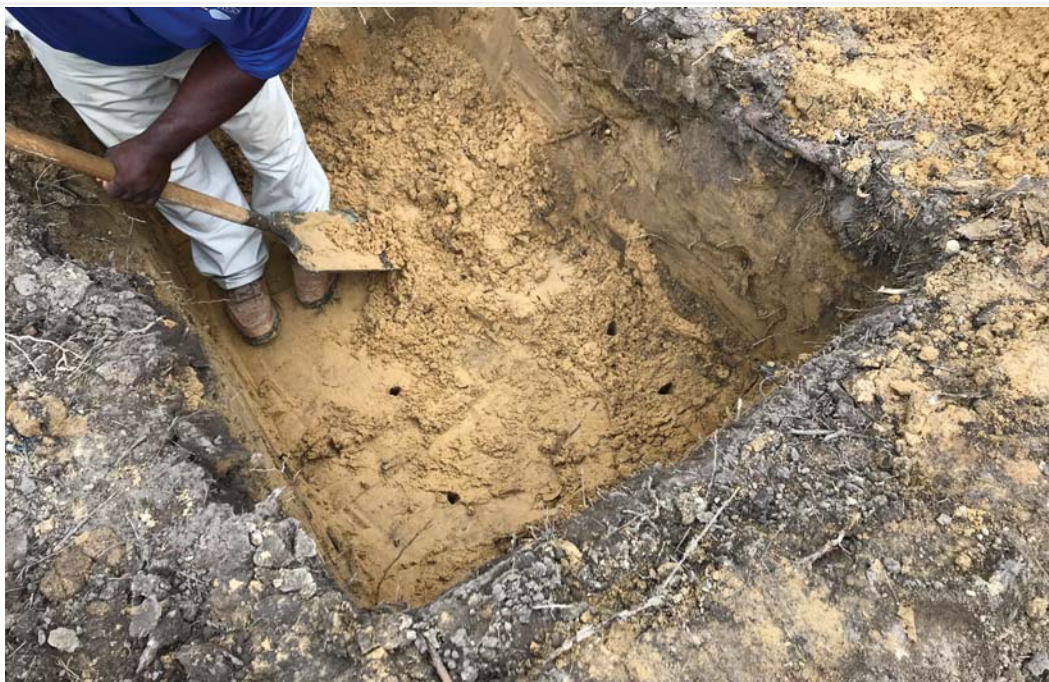
Site Conditions Observed
