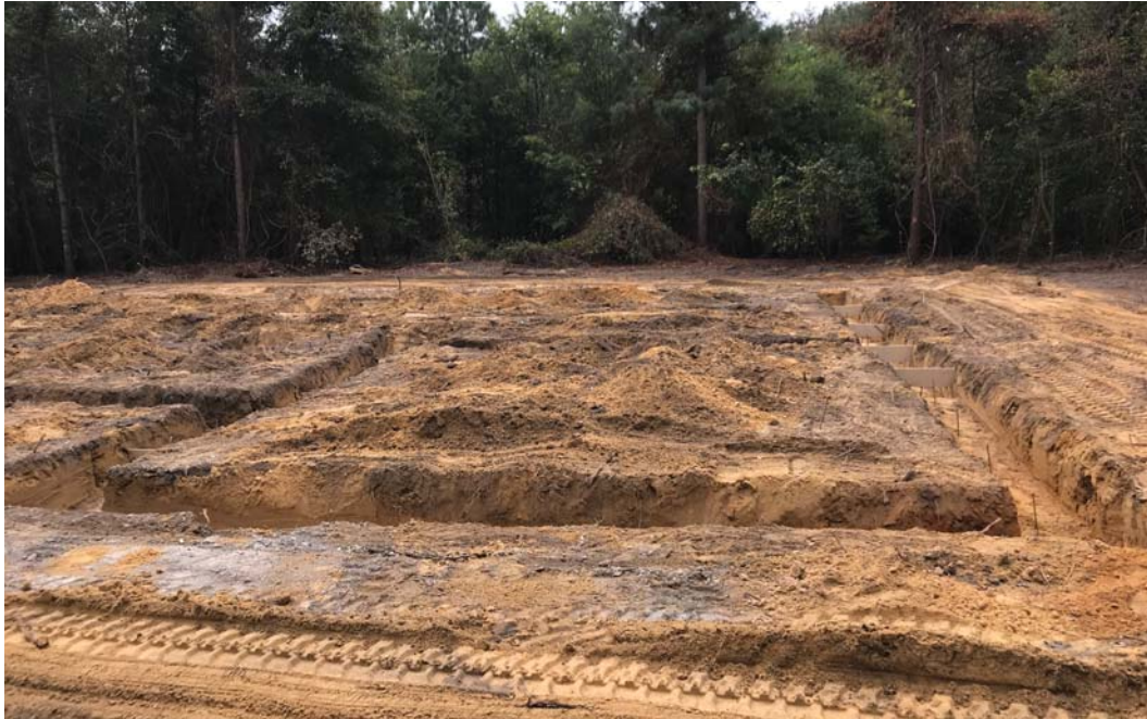
Site Conditions Observed
