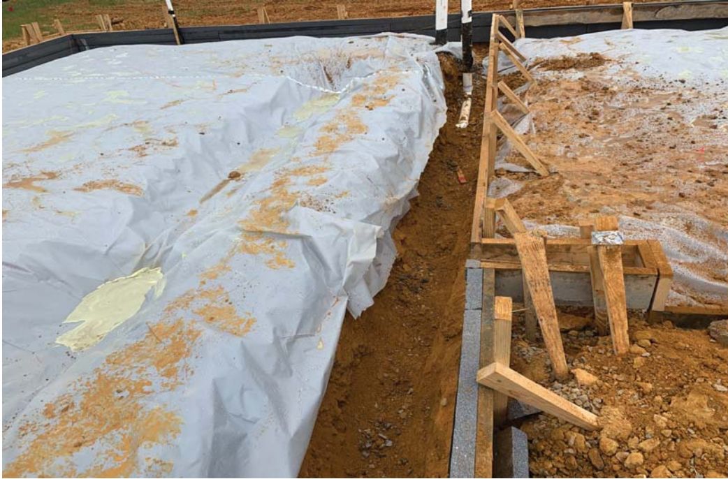
Site conditions observed - Lot 57
