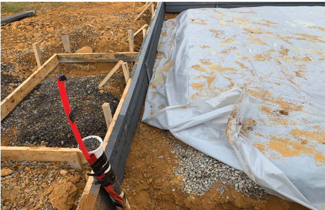
Site conditions observed - Lot 57
