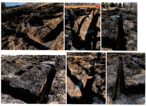
The footing soils were visually evaluated, probed with a  $\frac{1}{2}$ " rod and/or use of a DCP techniques to correlate surface soil conditions with bearing capacity. The area in the right rear of the building envelope had visible subsurface drainage. Rebar was added per instructions.
