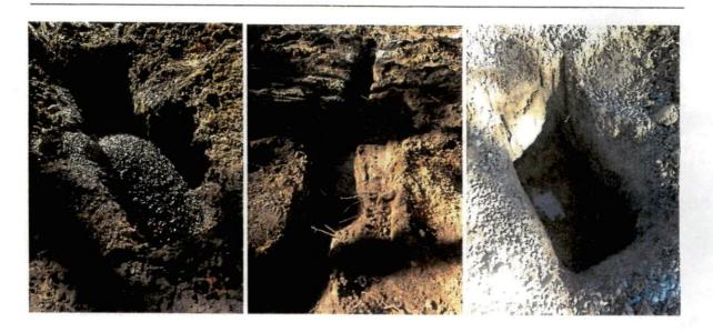
The footing trenches were partially complete into a combination of sandy soils with some organics. Trenches were completed under observation and soils beneath probed and visually graded.
