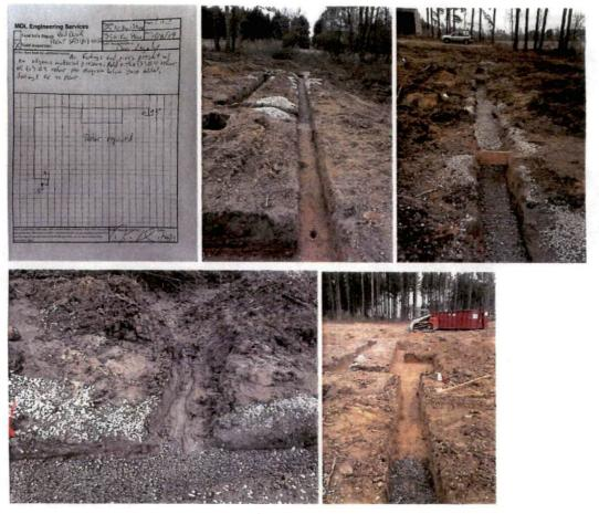
Organics, including root balls were discovered and removed down to virgin soil before filling with stone. The area in the right rear of the building envelope was excavated to approximately 5' depth and filled with washed stone.
