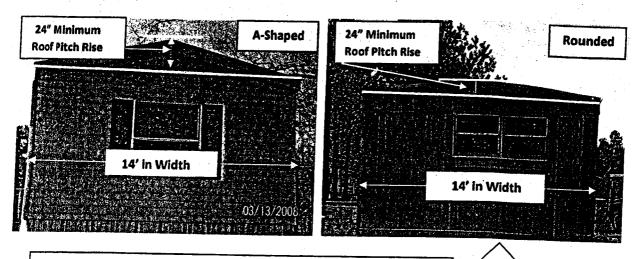
Note: Most Rounded Roofs **Will Not** Meet The Roof Pitch Requirement As Illustrated. The Measurement From The Peak Of The Roof To The Base Line Of The Roof Must Be 12" For Every 7' Of Total Width Of The Home. (Ex: 14' Wide Home = 24" Roof Rise)
