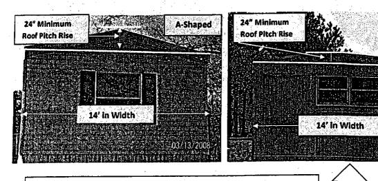
Note: Most Rounded Roofs Will Not Meet The Roof Pitch
