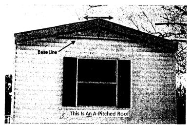
Measure Downward From The Center Of The Roof To The Base Line Of The Roof
