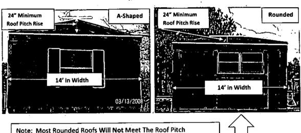
Note: Most Rounded Roofs Will Not Meet The Roof Pitch
