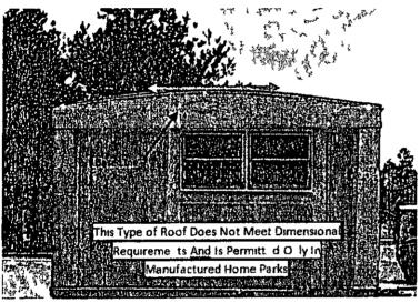
The Base Line Of The Roof Is Established By The Line Greated By Measuring Across The Home From Side To Side At The Edge Of The Roofing Material
