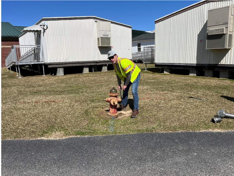
Photograph 1. Fire Hydrant (Flow Hydrant) located to the south of Lillington Shawtown Elementary, next to the mobile classrooms.
