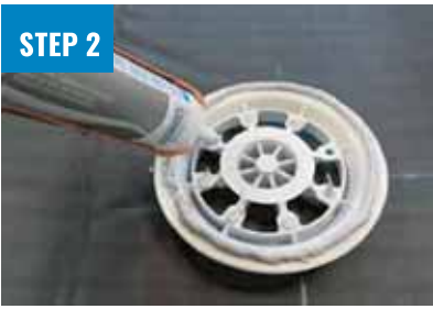
APPLY CHEMLINK M1 SEALANT
