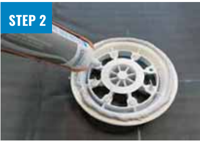
APPLY CHEMLINK M1 SEALANT
