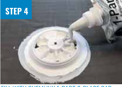
FILL WITH CHEMLINK 1-PART & PLACE CAP
