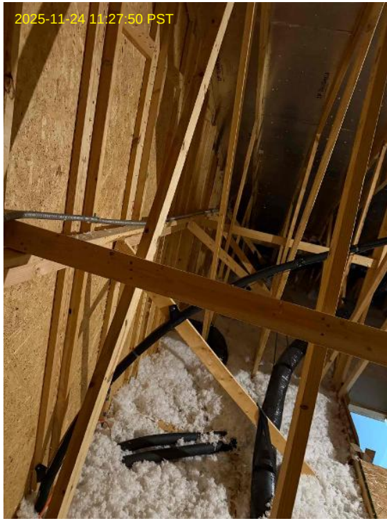
Internal Installers Loc: 35.6031, -78.8172
