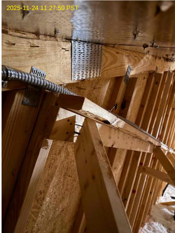
Internal Installers Loc: 35.6033, -78.8167
