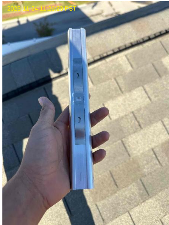
Roof Photos / Photo: Splice Bar
