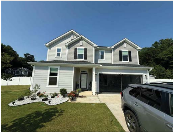
FRONT VIEW OF THE BUILDING
