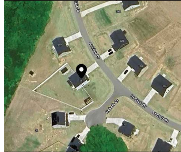
AERIAL VIEW OF THE BUILDING
