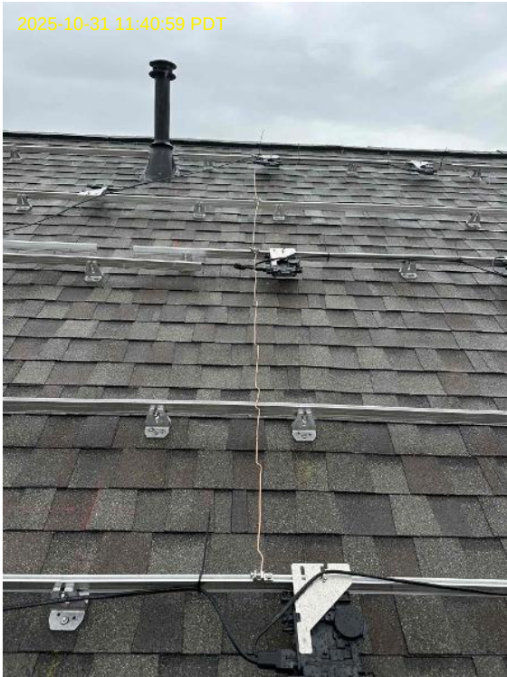
Roof Photos / Array 1 / Rail with Optos/Micros + EGC installed + Wire management
