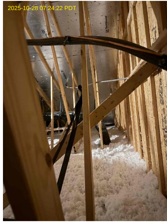
Internal Installers Loc: 35.4972, -78.809
