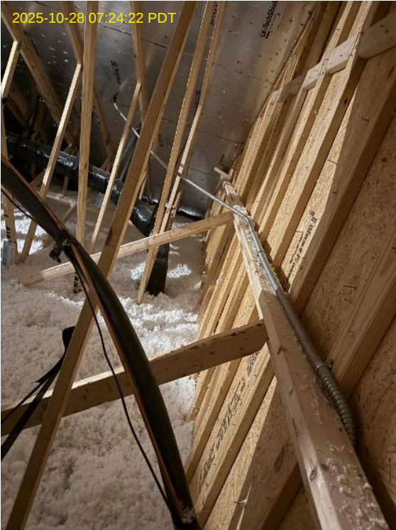
Internal Installers Loc: 35.4969, -78.8091
