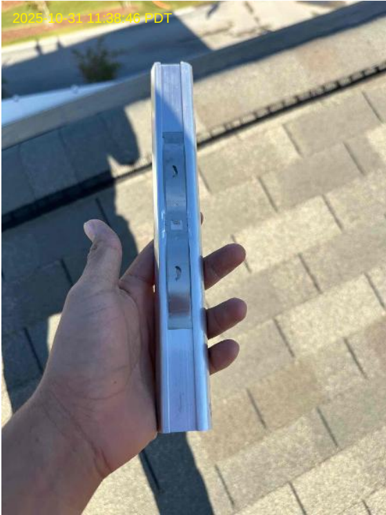
Roof Photos / Photo: Splice Bar
