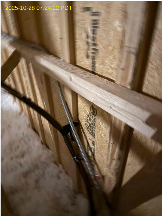
Internal Installers Loc: 35.4969, -78.8091
