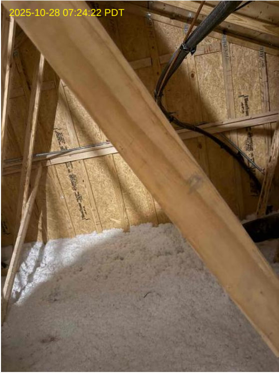
Internal Installers Loc: 35.4971, -78.809
