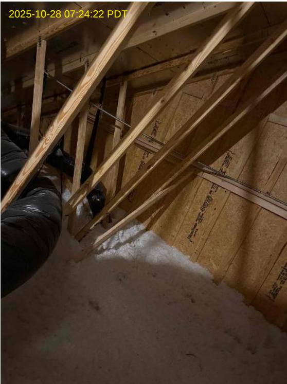
Internal Installers Loc: 35.4972, -78.809
