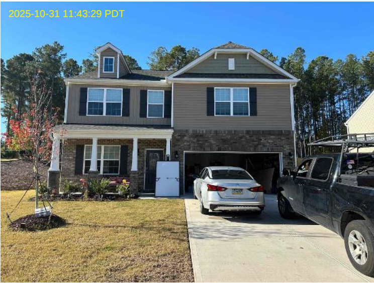
Component Identification / Photo of PV module in Front of Address
