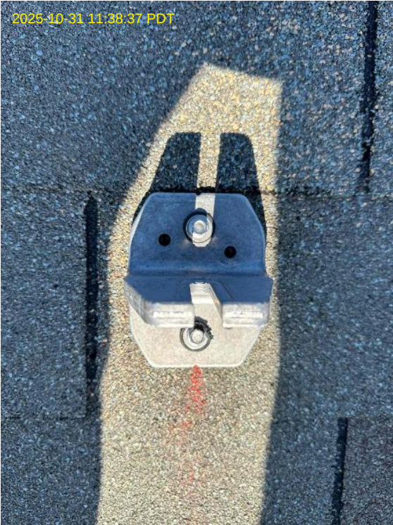
Roof Photos / Close up of attachment – Sealed & installed
