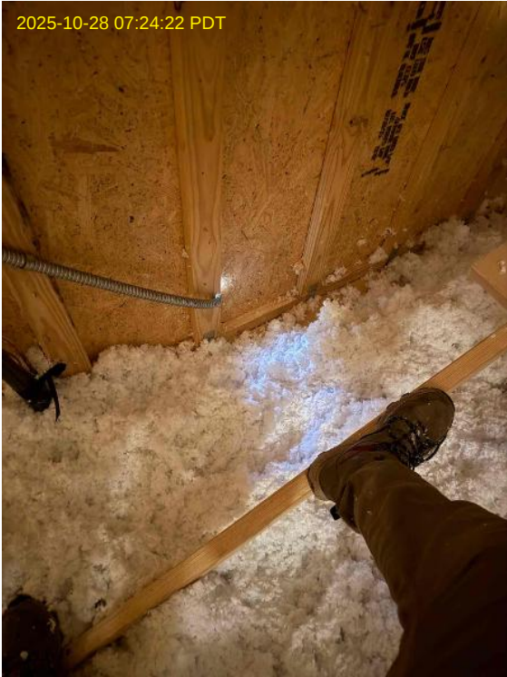
Internal Installers Loc: 35.497, -78.8091
