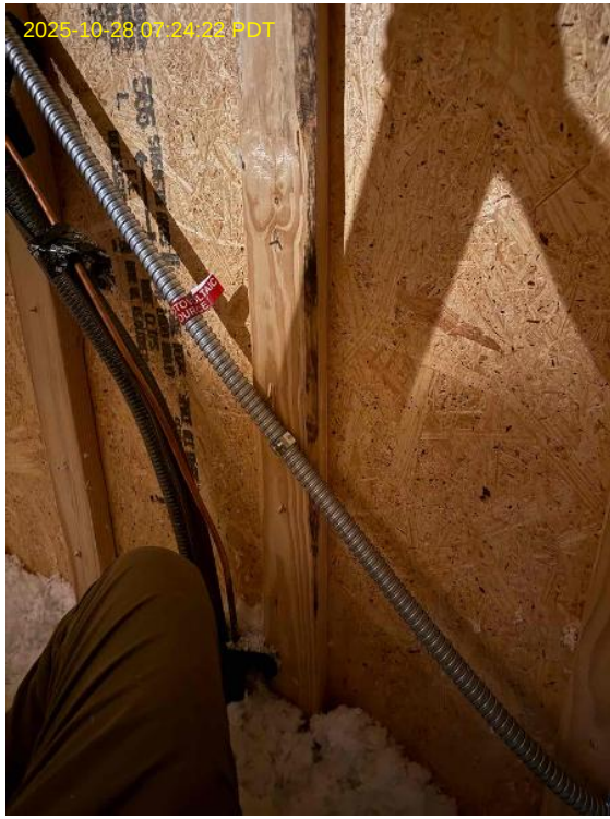
Internal Installers Loc: 35.497, -78.8091
