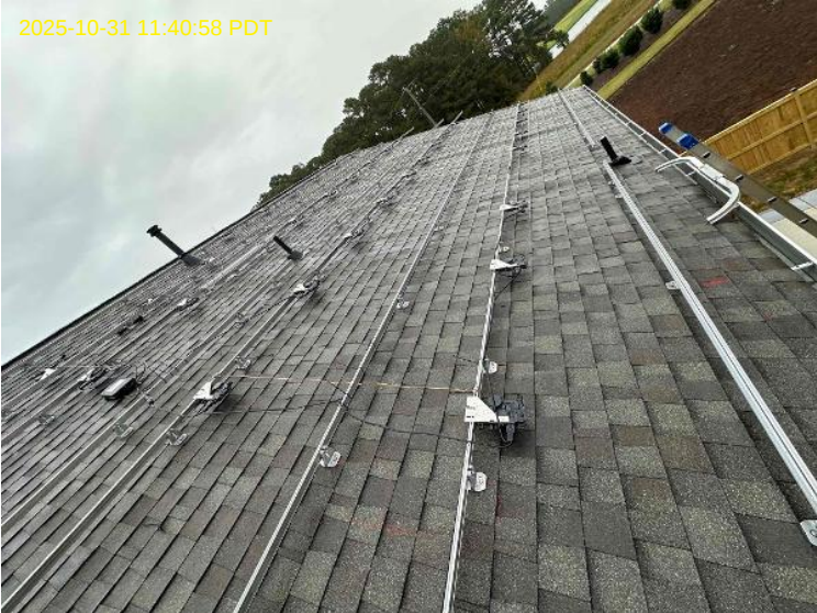
Roof Photos / Array 1 / Rail with Optos/Micros + EGC installed + Wire management
