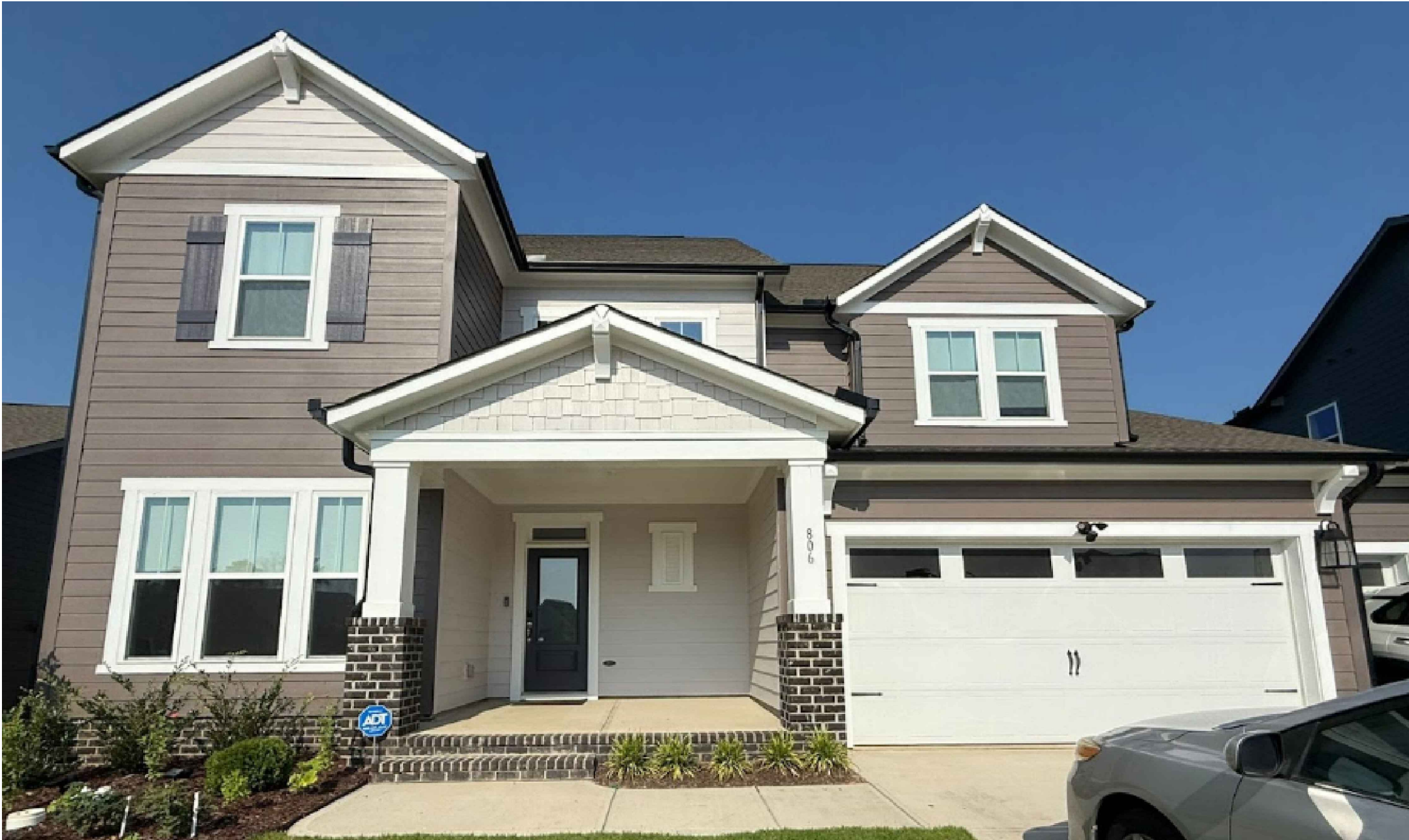
FRONT VIEW OF THE BUILDING
