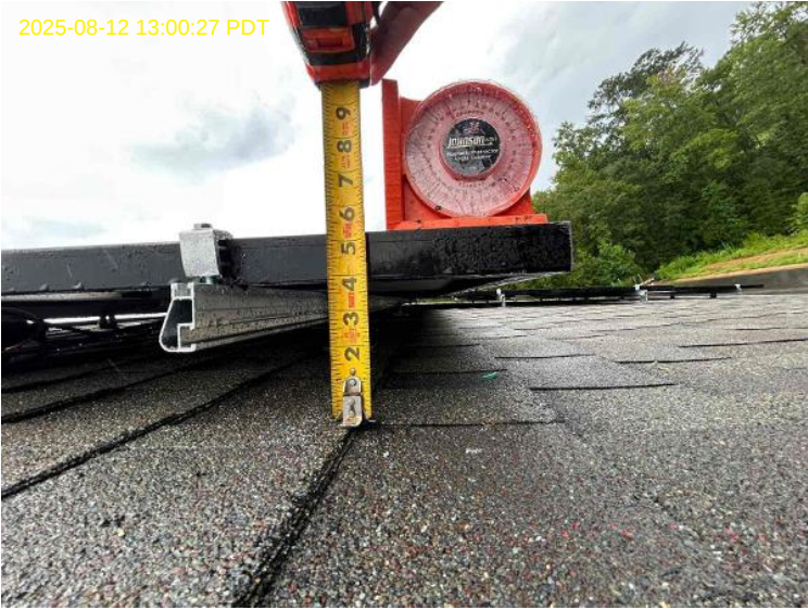
Roof Photos / Array 1 / Tilt - measured on array
