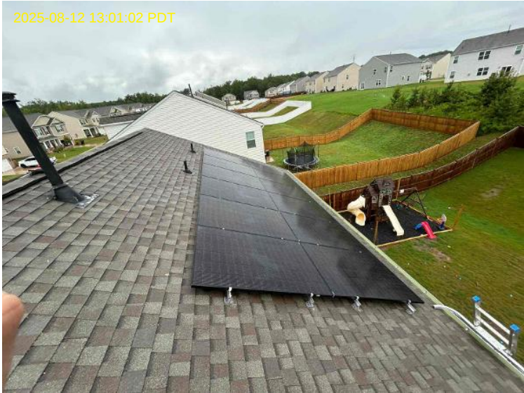
Roof Photos / Array 2 / Complete Array with all modules visible + Rail trimmed
