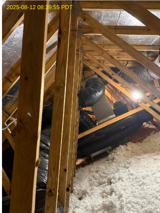
Internal Installers Loc: 35.5017, -78.8052
