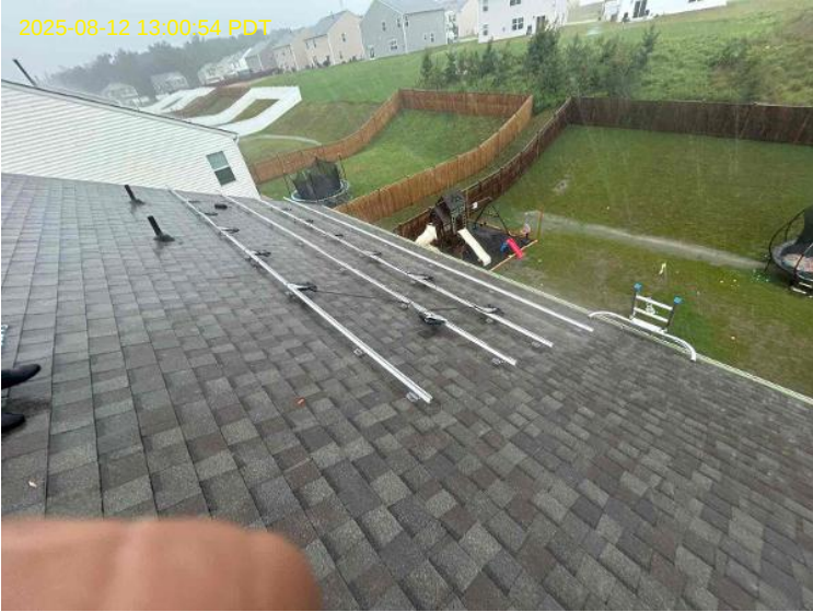
Roof Photos / Array 2 / Rail with Optos/Micros + EGC installed + Wire management
