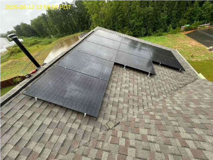
Roof Photos / Array 1 / Complete Array with all modules visible + Rail trimmed
