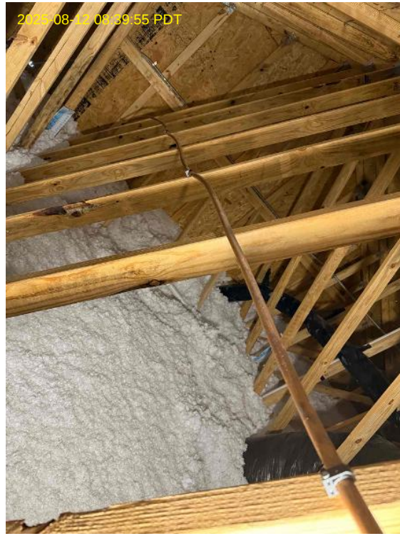
Internal Installers Loc: 35.5016, -78.8053
