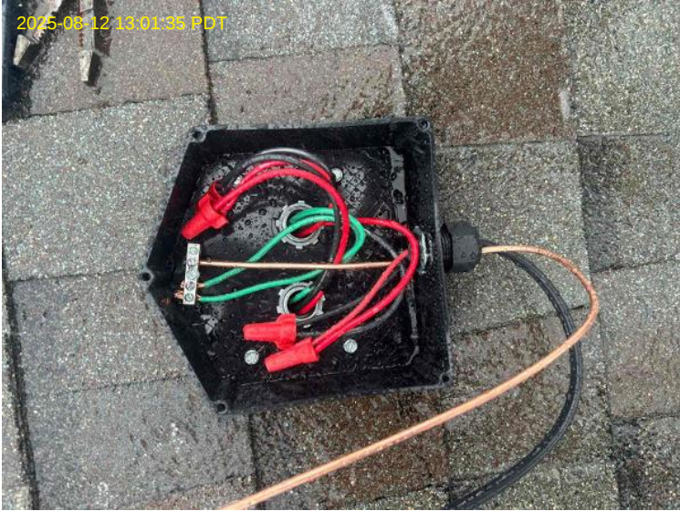
Roof Photos / Array 2 / Junction box - Internal wiring including terminations, bonding & grounding
