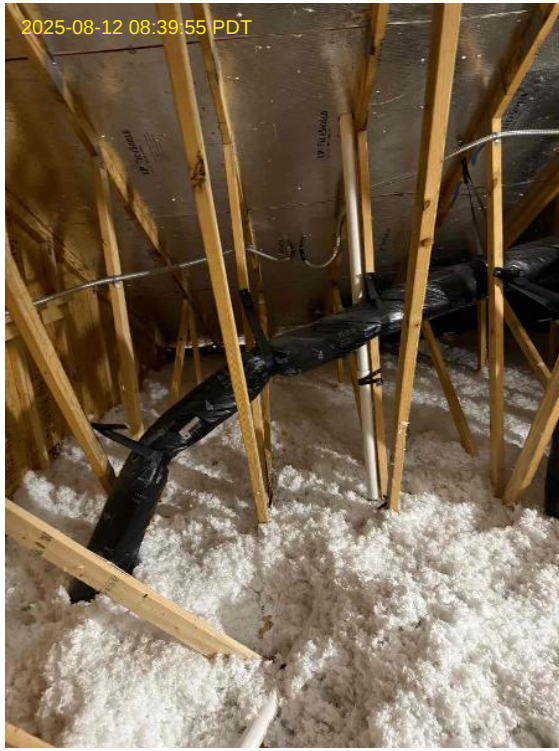
Internal Installers Loc: 35.5017, -78.8054
