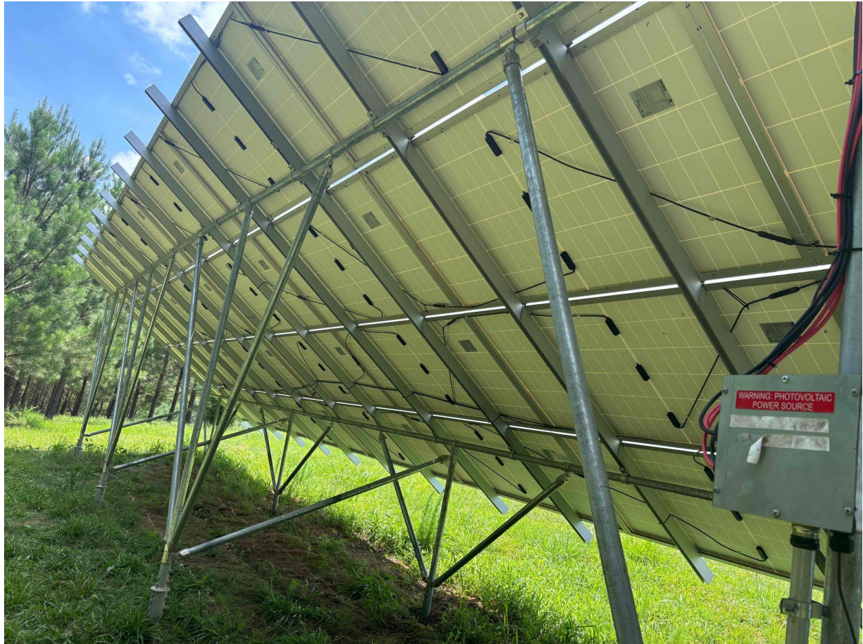
Inspection Photos: 2228 Buckhorn Rd, Sanford, NC 27330 (Krakowski)
