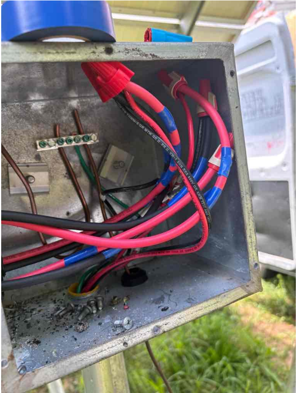
Inspection Photos: 2228 Buckhorn Rd, Sanford, NC 27330 (Krakowski)
