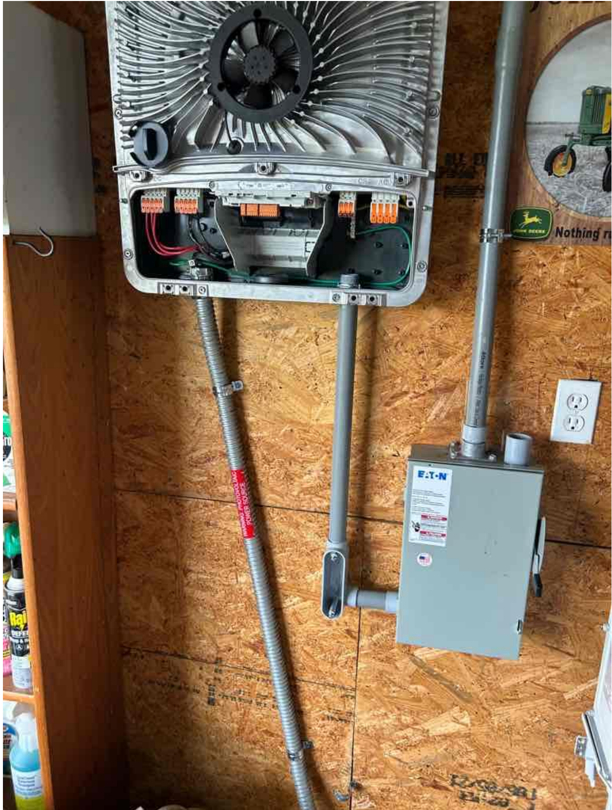
Inspection Photos: 2228 Buckhorn Rd, Sanford, NC 27330 (Krakowski)
