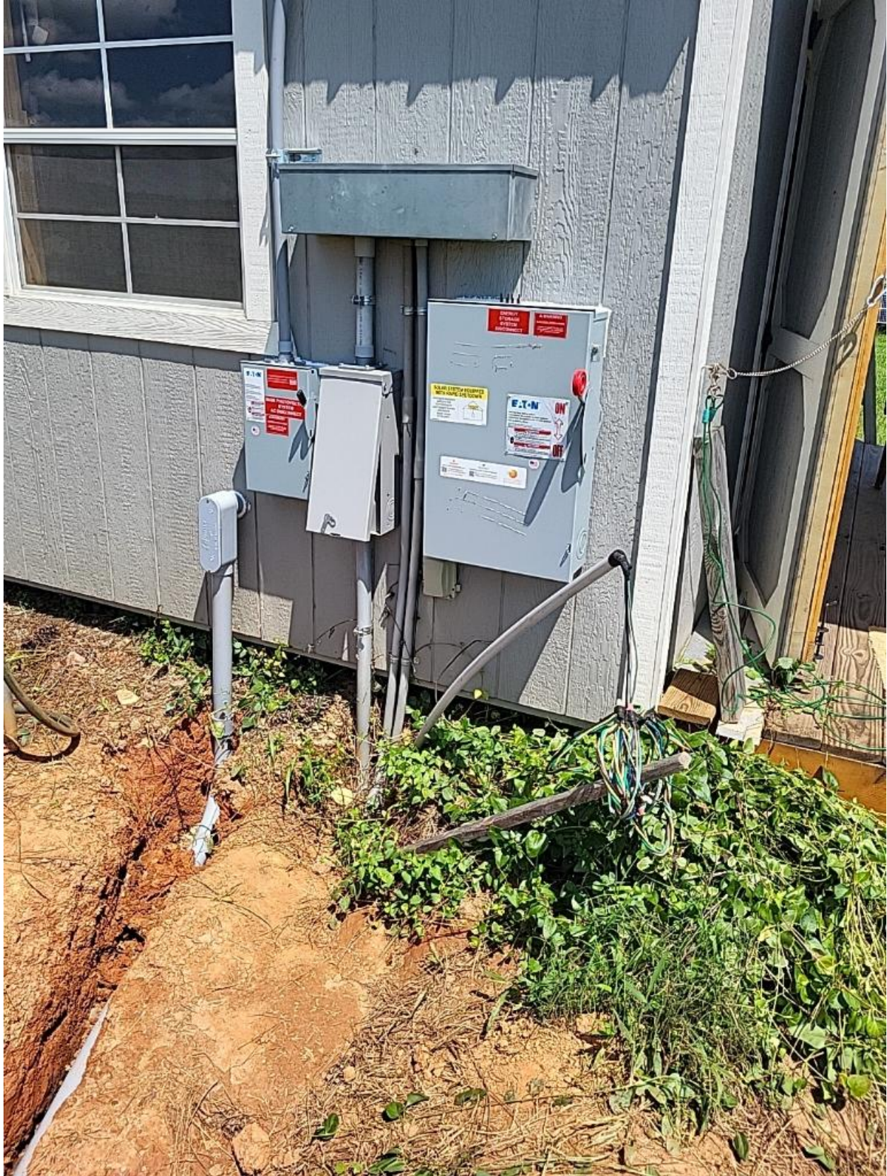
Inspection Photos: 2228 Buckhorn Rd, Sanford, NC 27330 (Krakowski)
