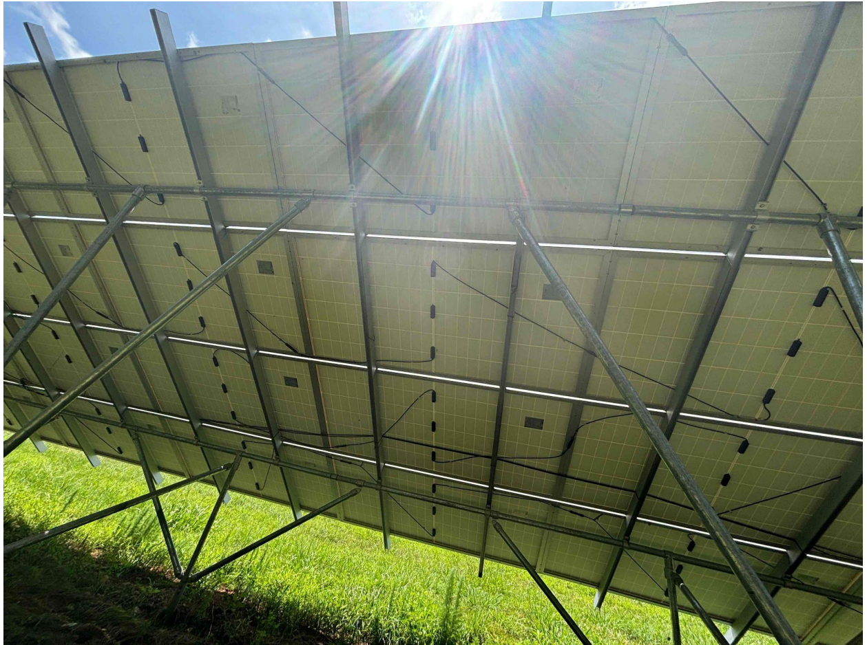
Inspection Photos: 2228 Buckhorn Rd, Sanford, NC 27330 (Krakowski)
