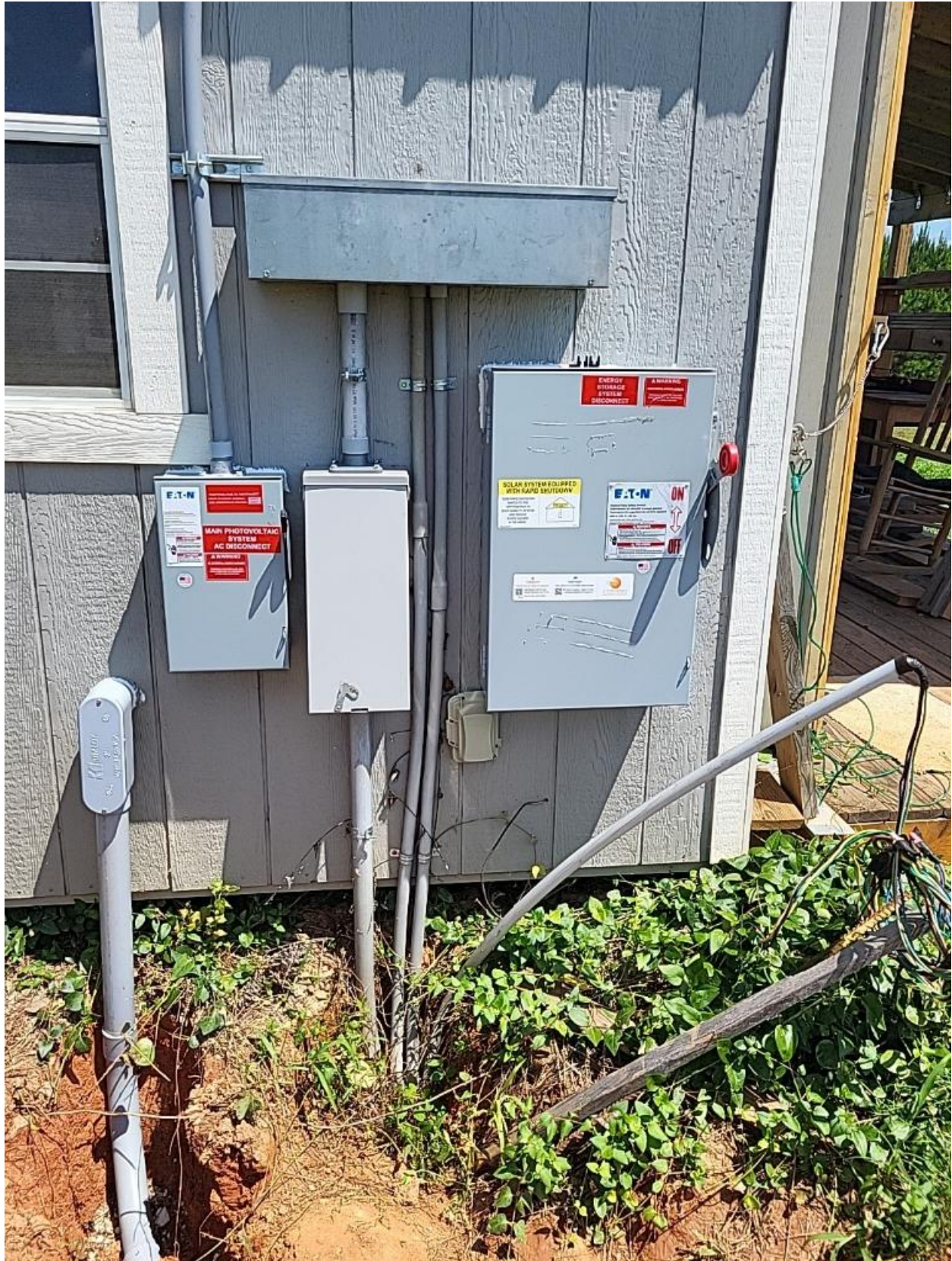
Inspection Photos: 2228 Buckhorn Rd, Sanford, NC 27330 (Krakowski)
