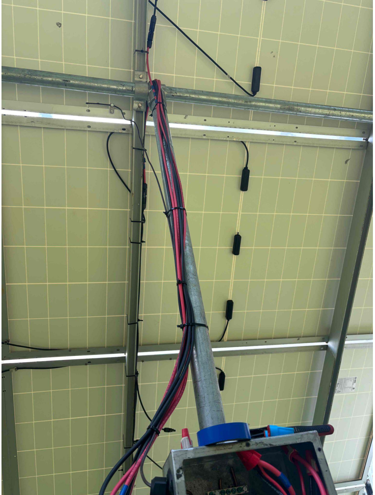
Inspection Photos: 2228 Buckhorn Rd, Sanford, NC 27330 (Krakowski)
