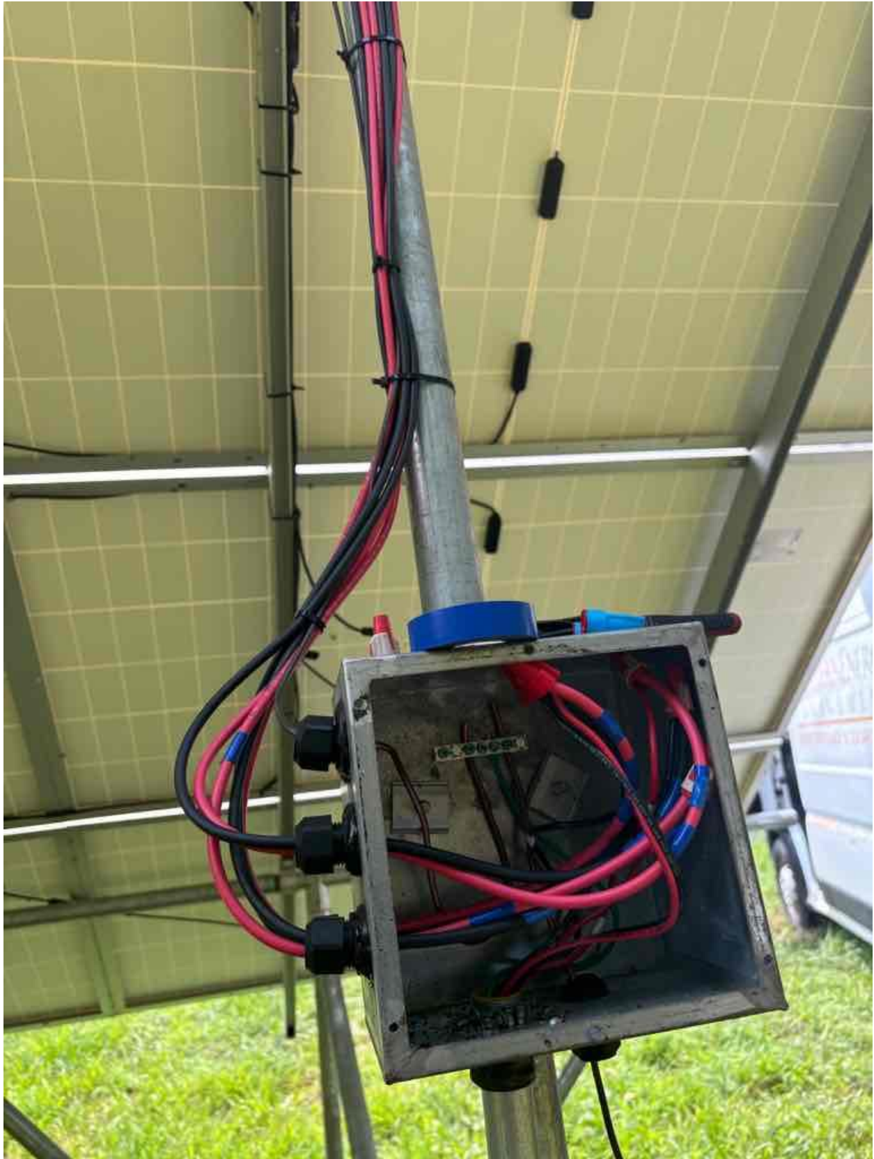
Inspection Photos: 2228 Buckhorn Rd, Sanford, NC 27330 (Krakowski)
