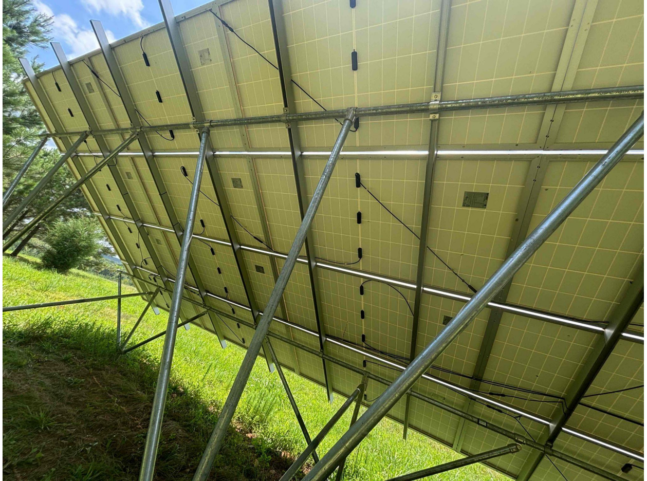
Inspection Photos: 2228 Buckhorn Rd, Sanford, NC 27330 (Krakowski)
