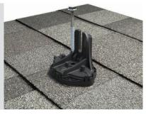
**4**Drive the lag until the InstaFlash is fully seated to the roof.
