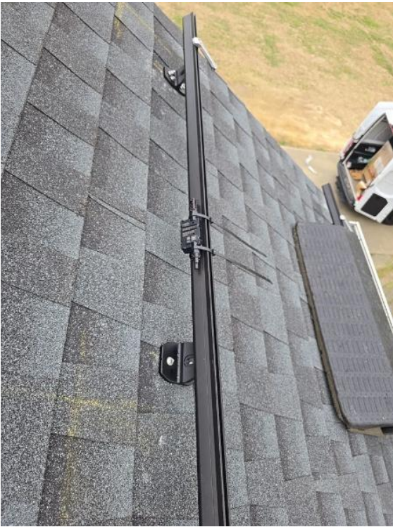
Roof / Rapid Shut Downs - Roof run
