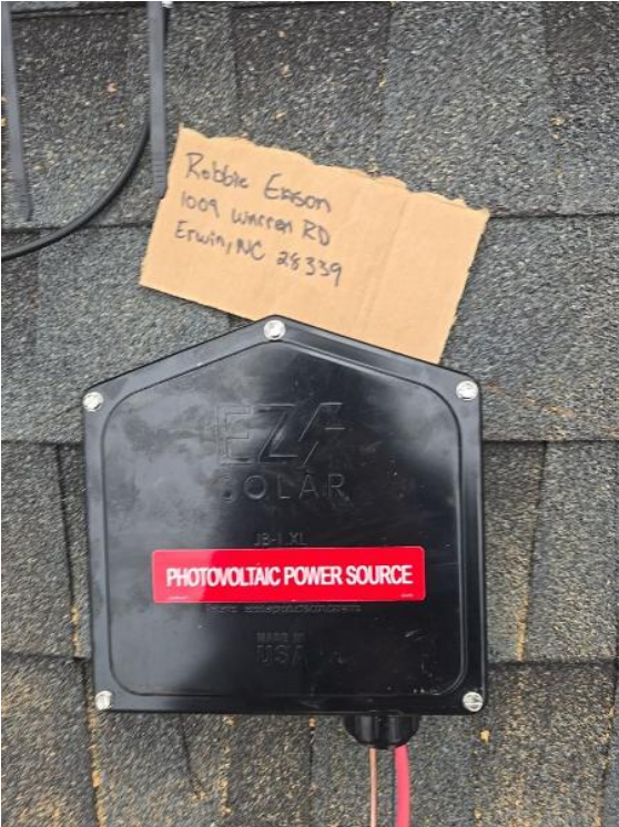
Roof / Soladeck with Lid On
