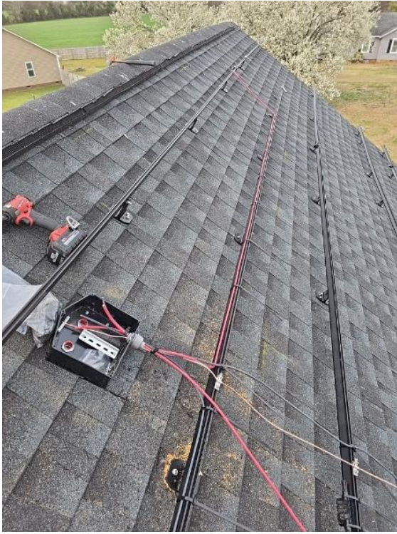
Roof / Wire Runs on roof
