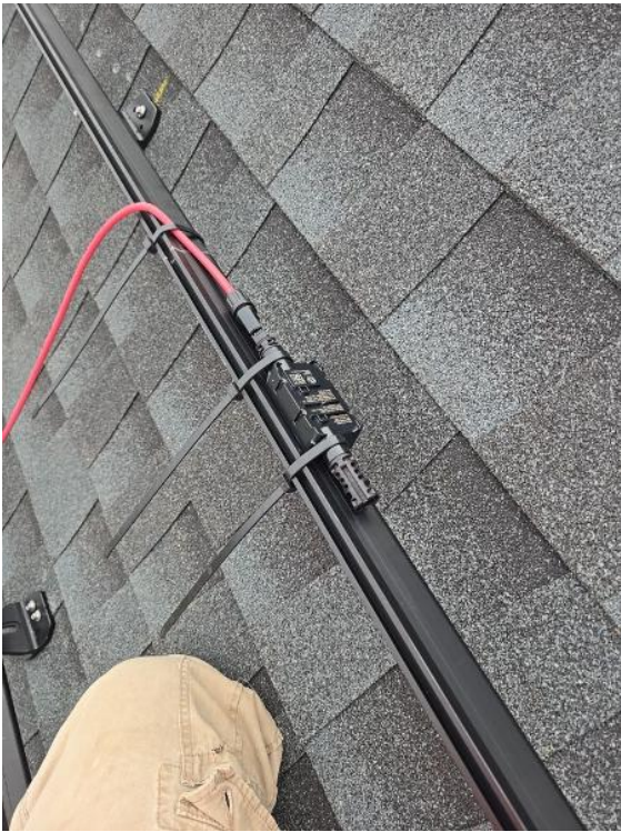
Roof / Rapid Shut Downs - Roof run
