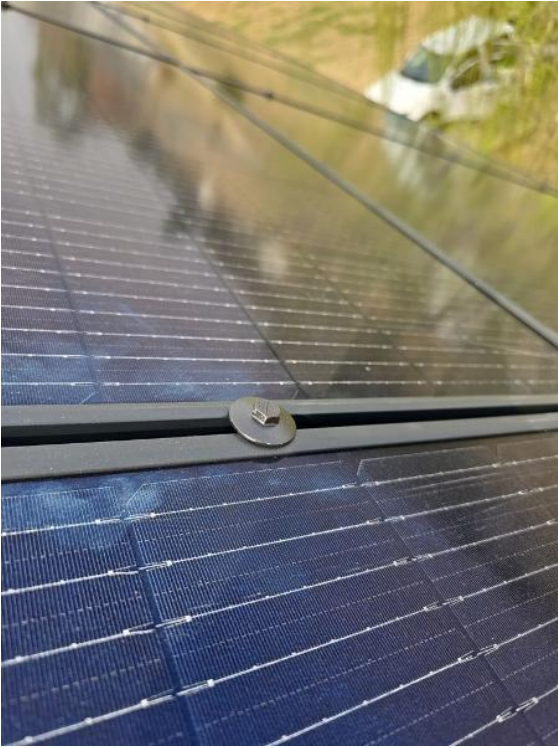
Roof / Mids - Installed (Up close)
