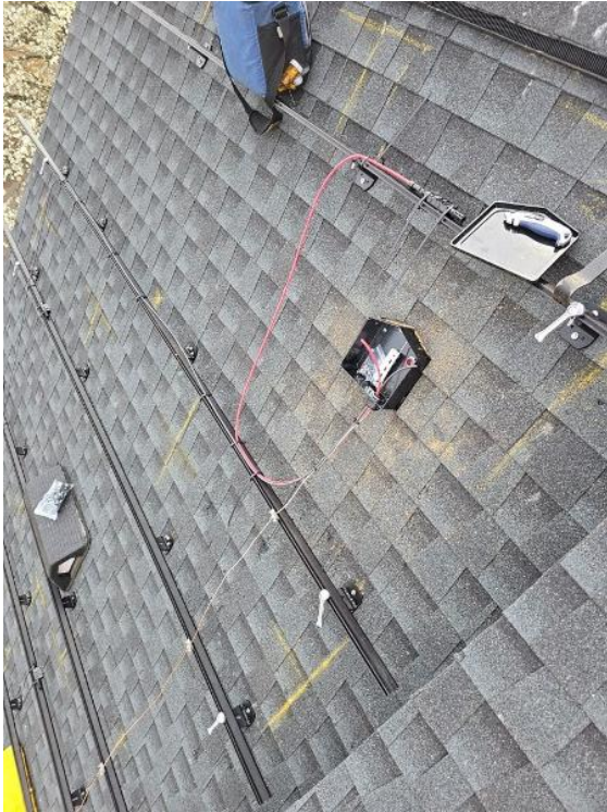
Roof / Wire Runs on roof
