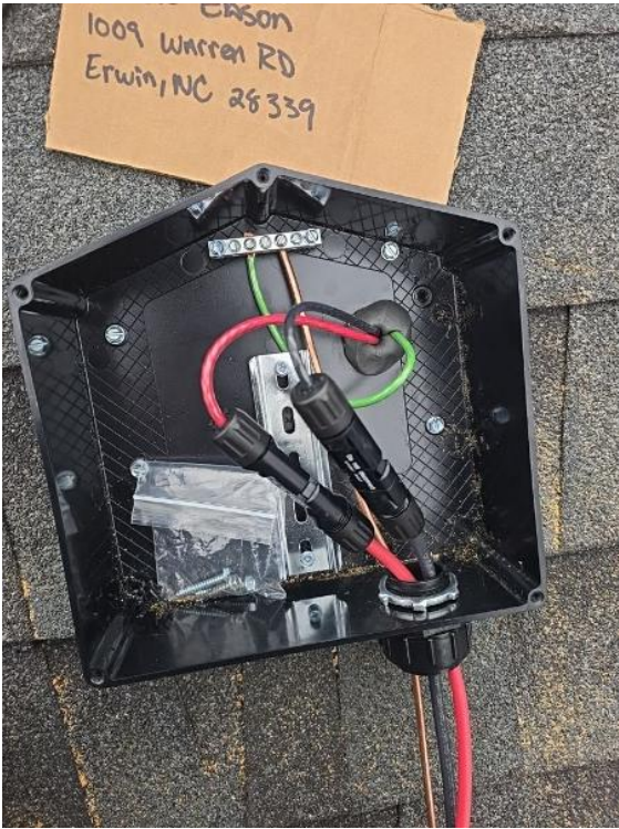
Roof / Soladeck showing all wiring connections
