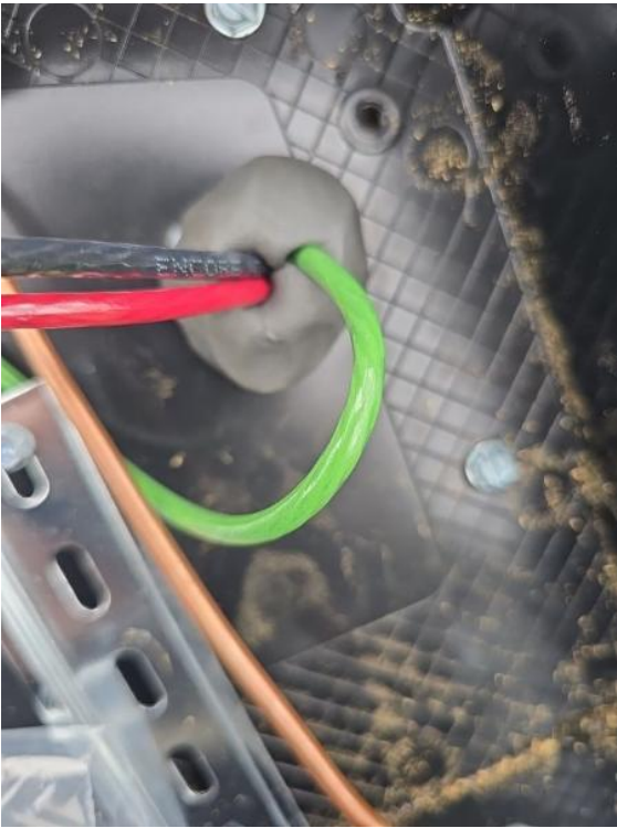
Roof / Duct seal in soladeck
