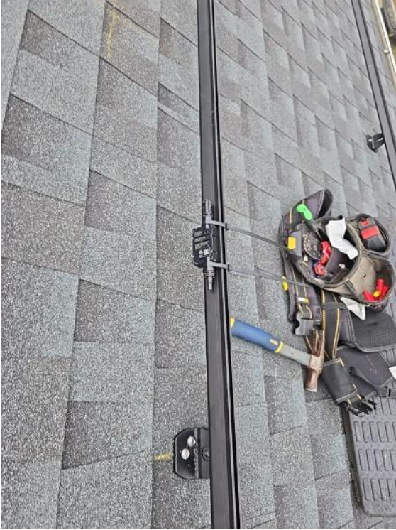
Roof / Rapid Shut Downs - Roof run
