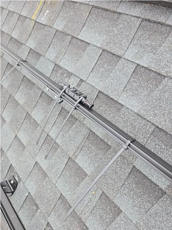
Roof / Rapid Shut Downs - Roof run
