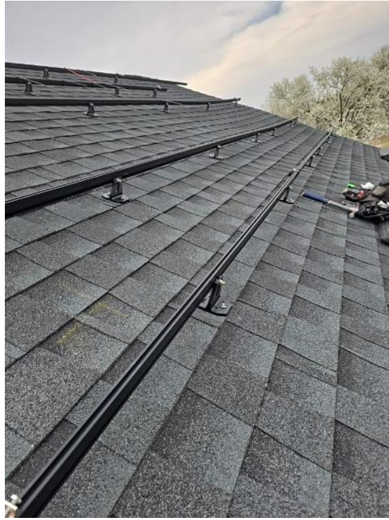
Roof / Rail Mounts - Roof Run
