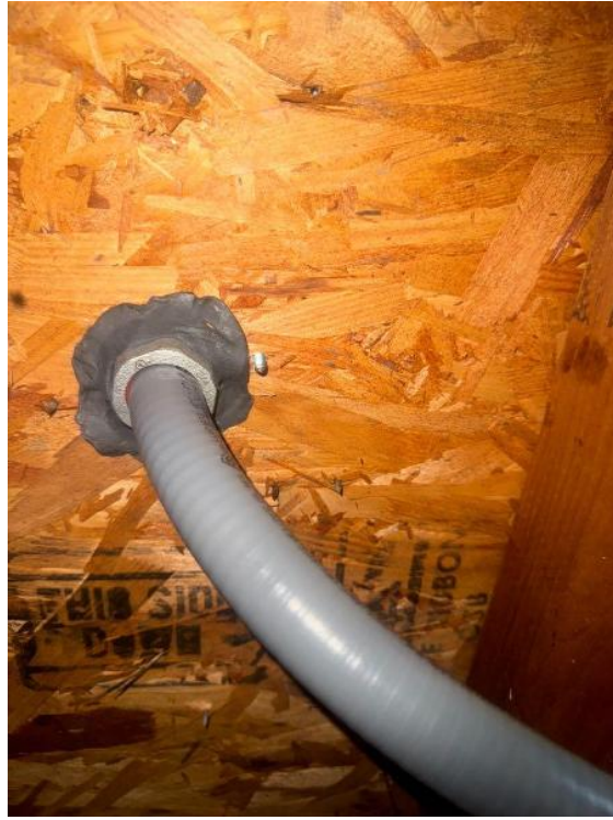
Attic / Sealed entry point
