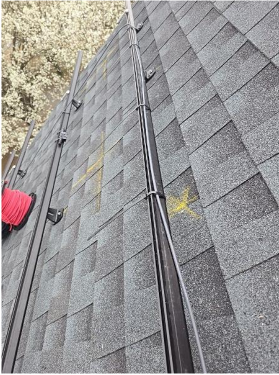
Roof / Roof Wiring at Rail
