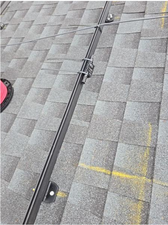
Roof / Rapid Shut Downs - Roof run
