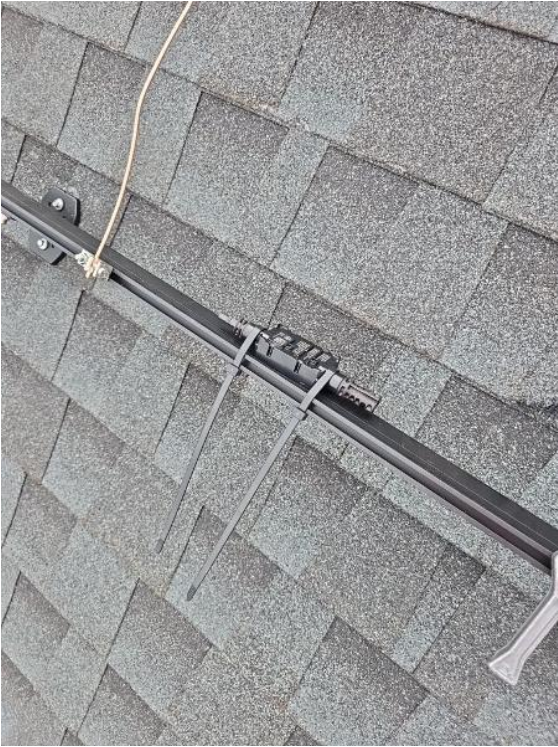
Roof / Rapid Shut Downs - Roof run
