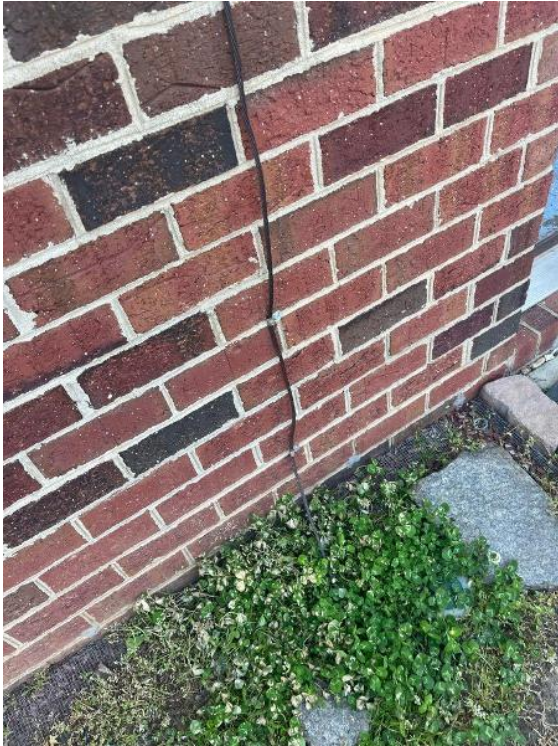
Electrical Equipment / Ground wire
