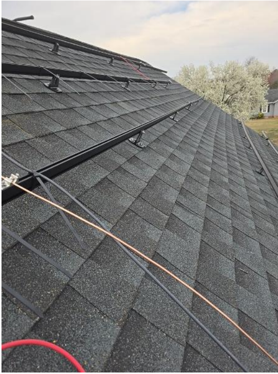
Roof / Rail Mounts - Roof Run
