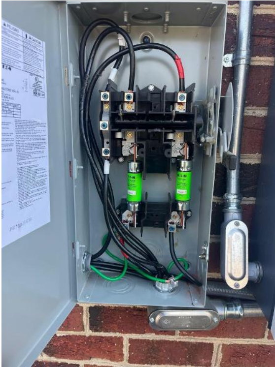
Electrical Equipment / Disconnect - With cover open
