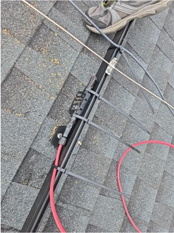
Roof / Rapid Shut Downs - Roof run
