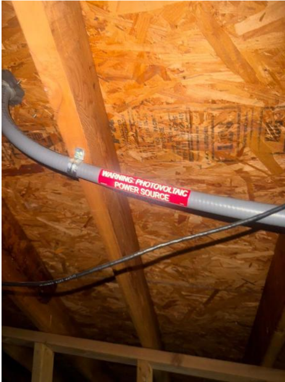
Attic / Attic conduit runs (3-4 images)
