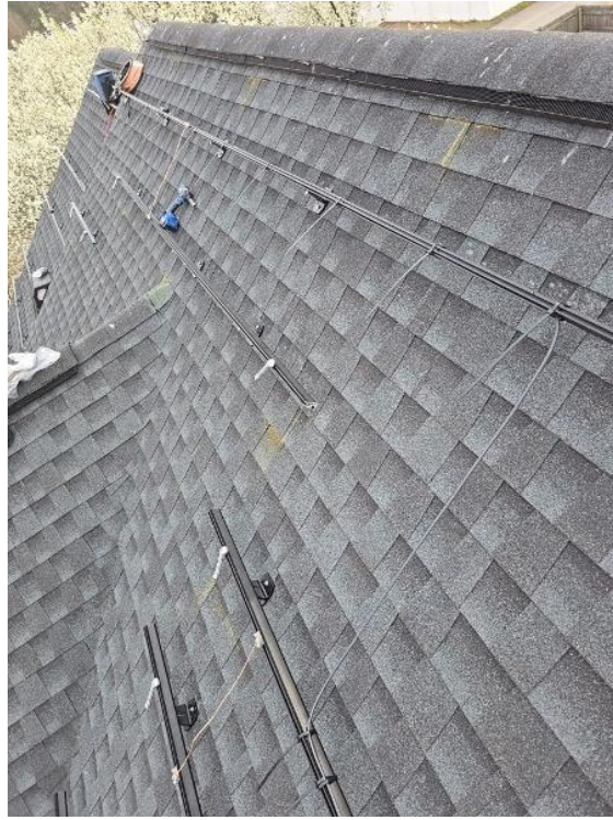
Roof / Wire Runs on roof
