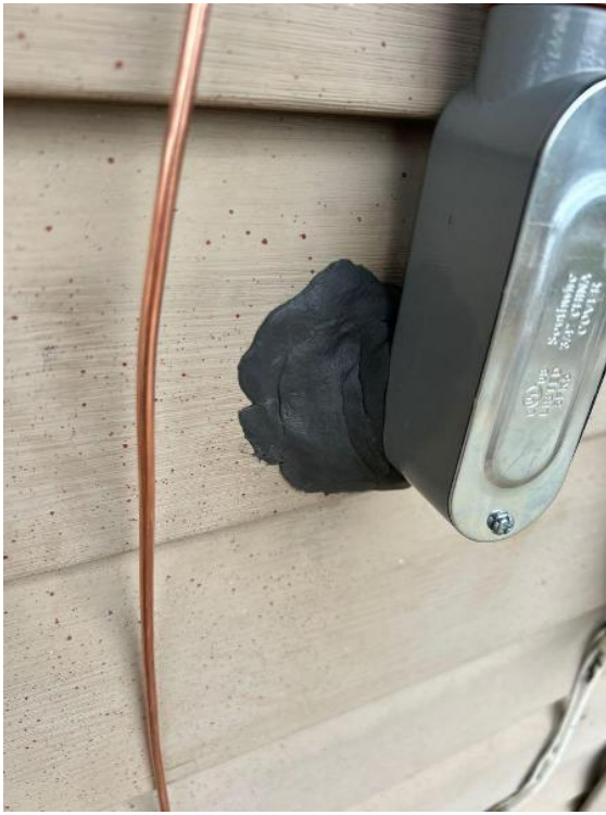
Electrical Equipment / Sealing of LB above 8ft
