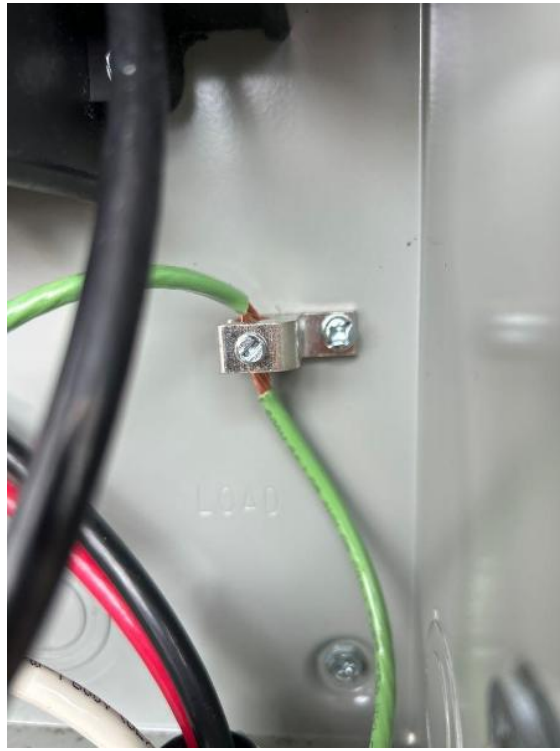
Electrical Equipment / Ground lug inside Disconnect
