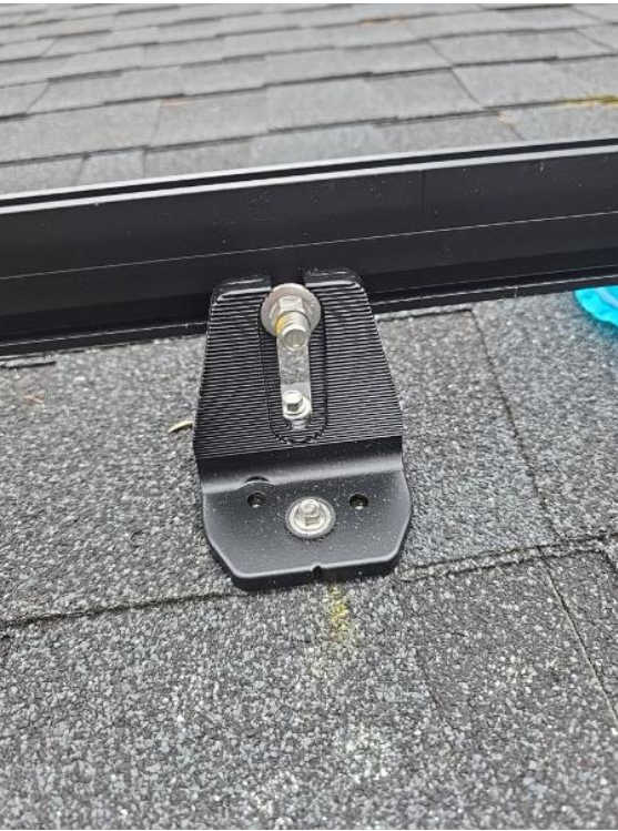
Roof / Rail Mounts (close up)
