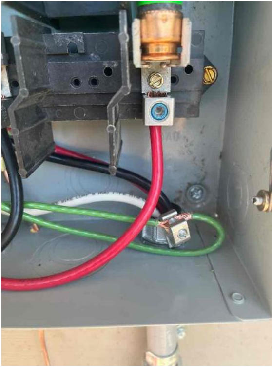
Electrical Equipment / Bonding Bushing in AC disconnect (2)
