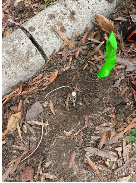
Electrical Equipment / Ground Rod
