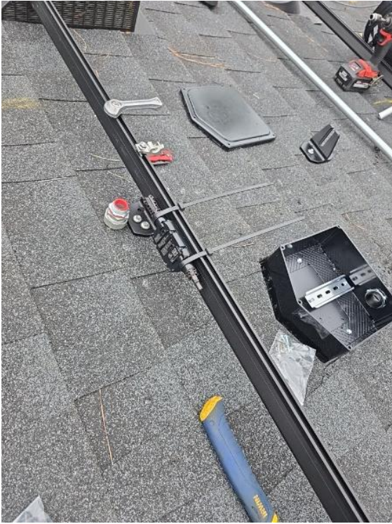
Roof / Rapid Shut Downs - Roof run
