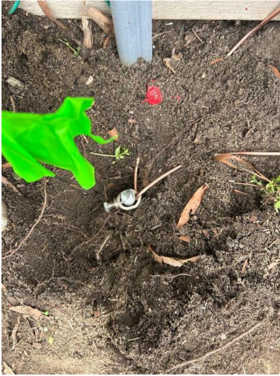
Electrical Equipment / Ground Rod
