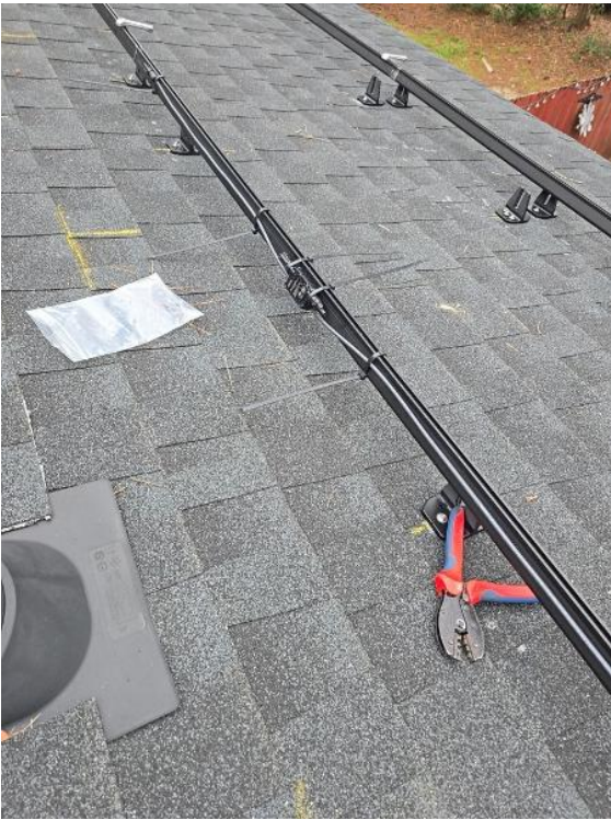
Roof / Rapid Shut Downs - Roof run
