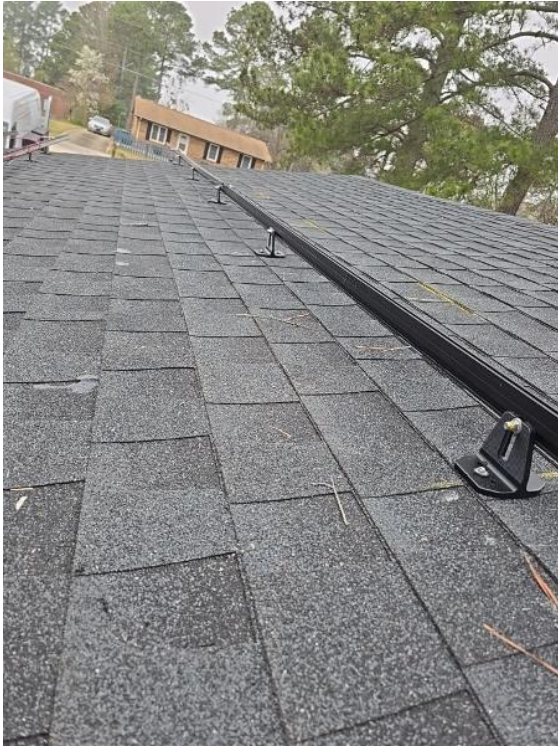
Roof / Rail Mounts - Roof Run
