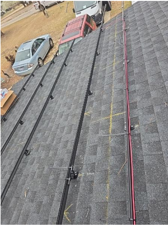
Roof / Rapid Shut Downs - Roof run
