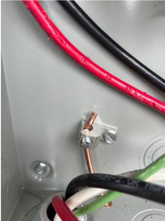
Electrical Equipment / Ground lug inside Disconnect
