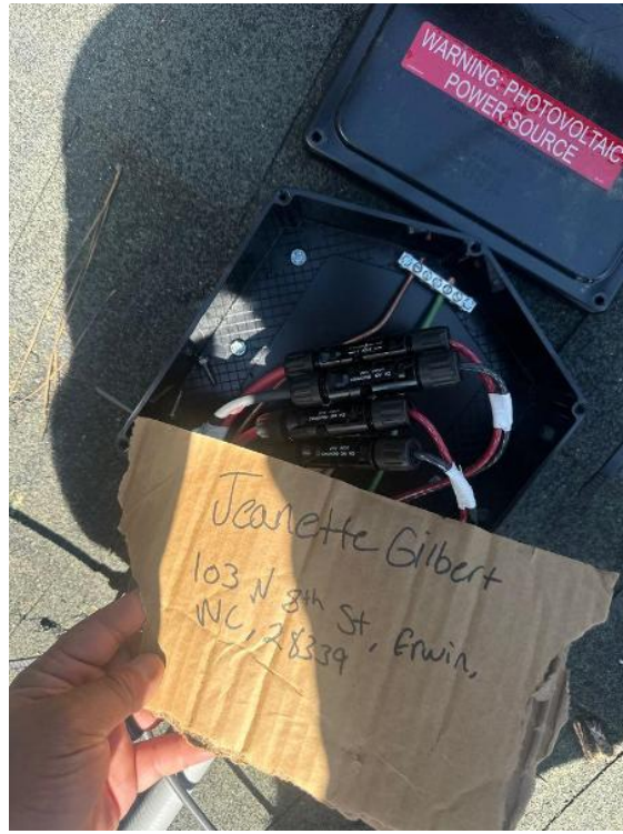
Roof / Soladeck showing all wiring connections
