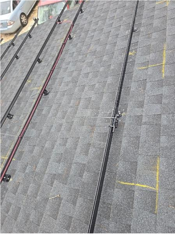
Roof / Rapid Shut Downs - Roof run
