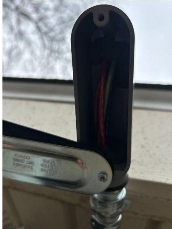
Electrical Equipment / Sealing of LBs, LLs, and LRs at mounted equipment
