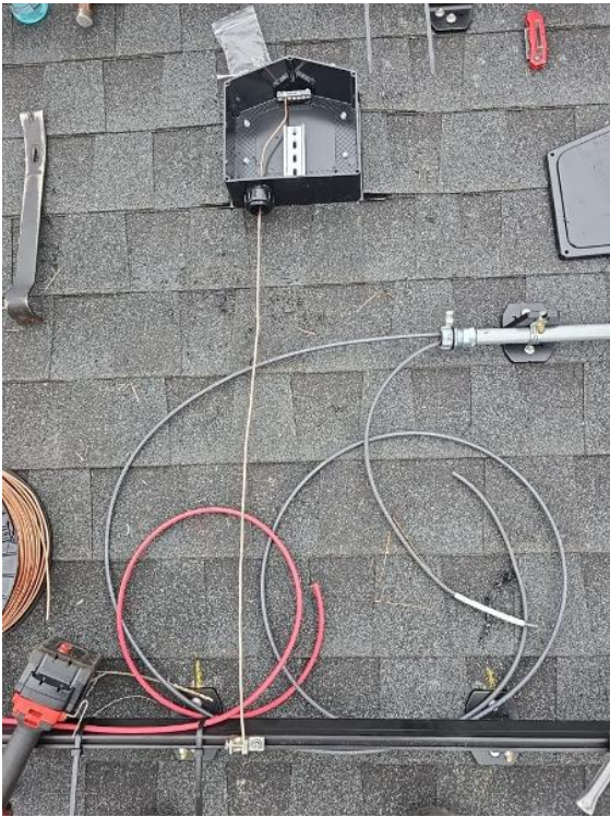
Roof / Grounding Connection between rails at each array
