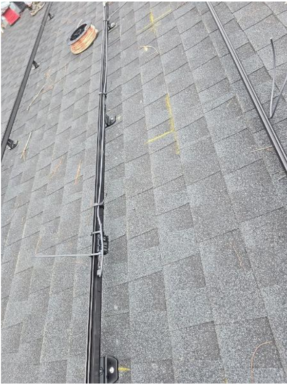
Roof / Rapid Shut Downs - Roof run
