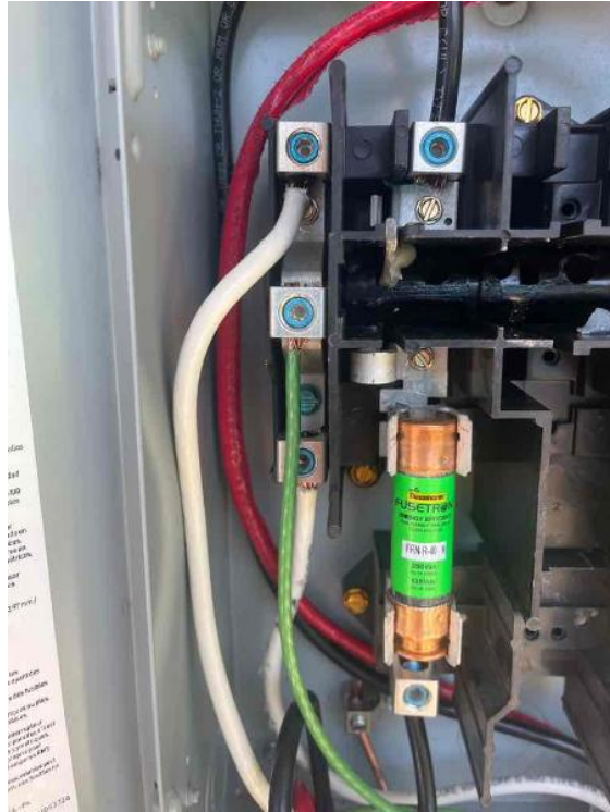
Electrical Equipment / Ground lug inside Disconnect
