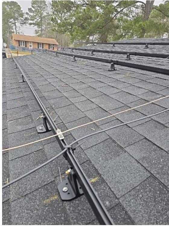
Roof / Rail Mounts - Roof Run
