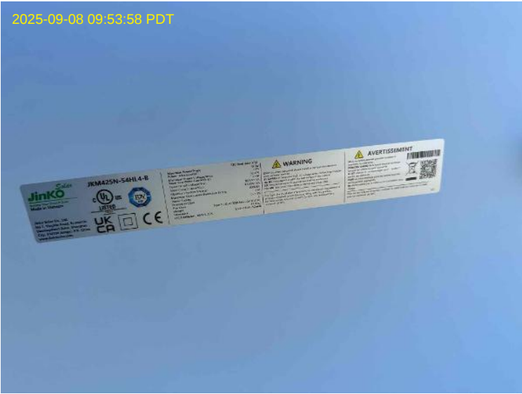
Component Identification / PV Module data label - Pull back of panel label on site
