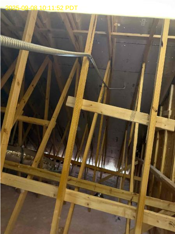
Internal Installers Loc: 35.4713, -78.8128
