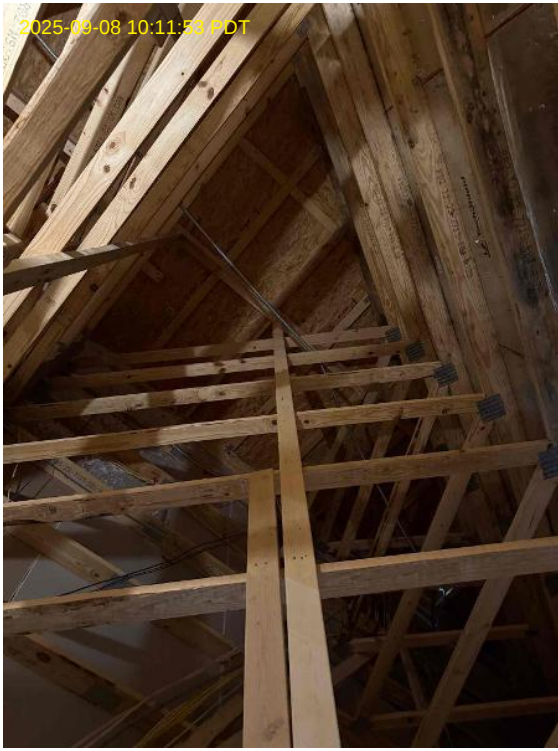
Internal Installers Loc: 35.471, -78.8127
