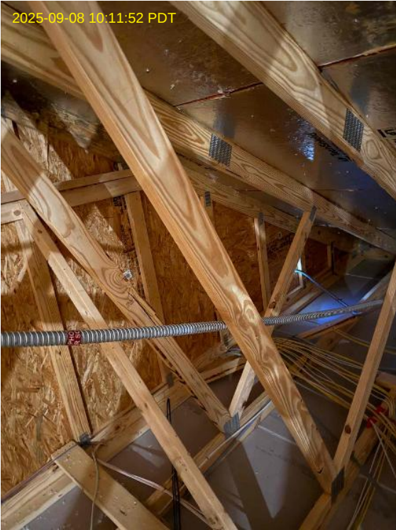
Internal Installers Loc: 35.4712, -78.813
