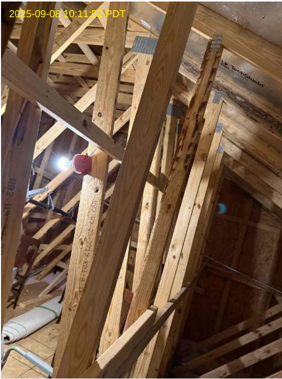
Internal Installers Loc: 35.4711, -78.8127
