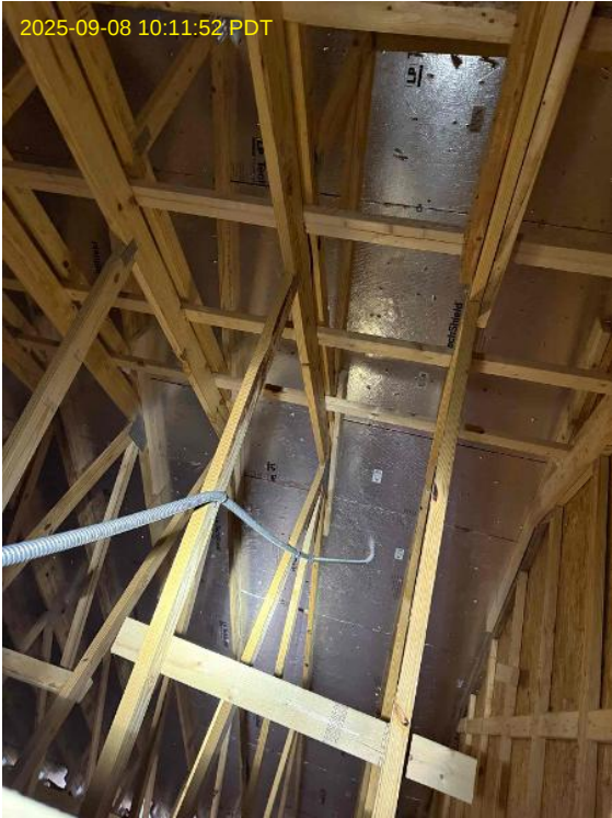
Internal Installers Loc: 35.471, -78.8129
