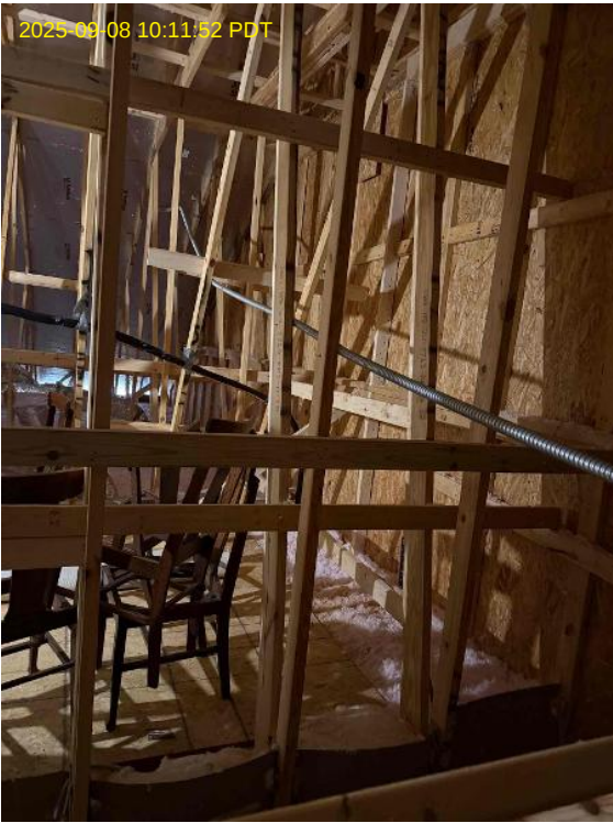
Internal Installers Loc: 35.4712, -78.813
