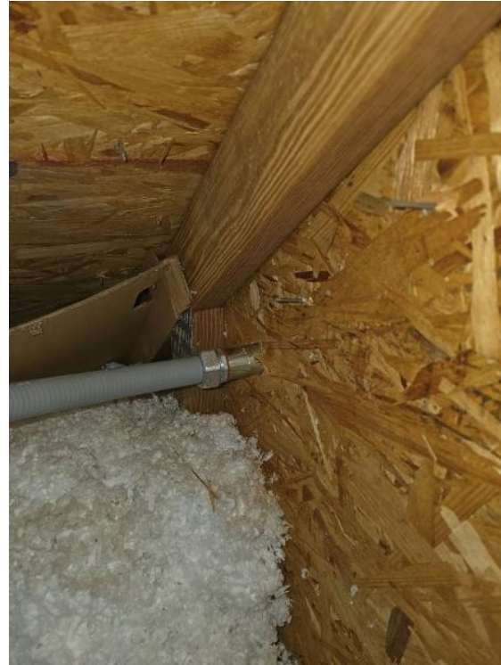
Attic / Entry point of conduit
