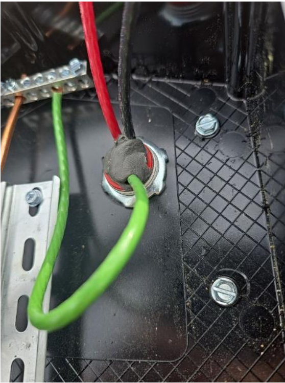
Roof / Duct seal in soladeck
