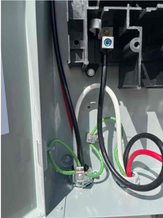
Electrical Equipment / Ground lug inside Disconnect
