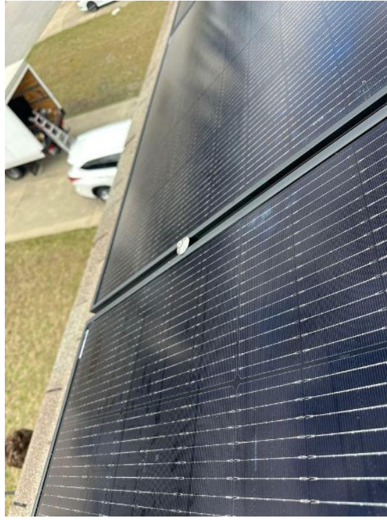
Roof / Mids - Installed (Up close)
