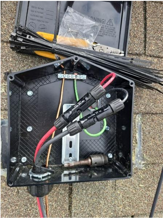
Roof / Soladeck showing all wiring connections
