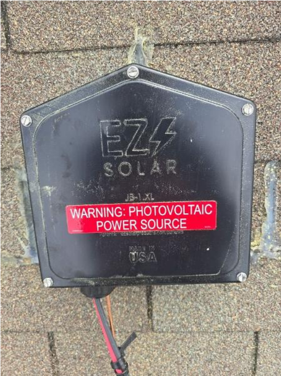
Roof / Soladeck with Lid On
