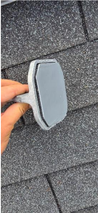
Roof / Sealing around L feet
