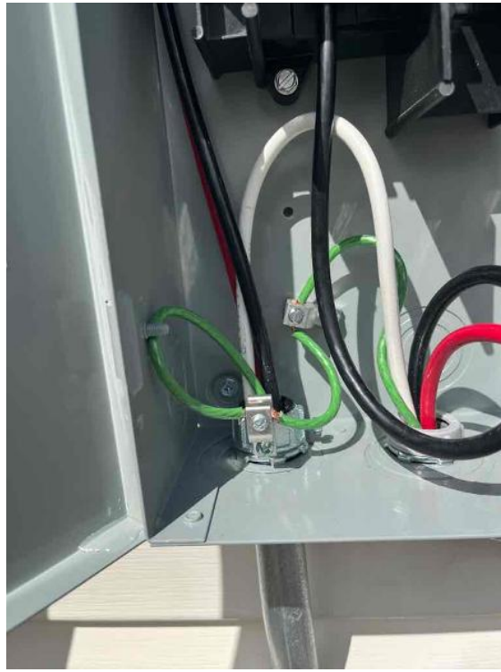
Electrical Equipment / Bonding Bushing in AC disconnect (2)
