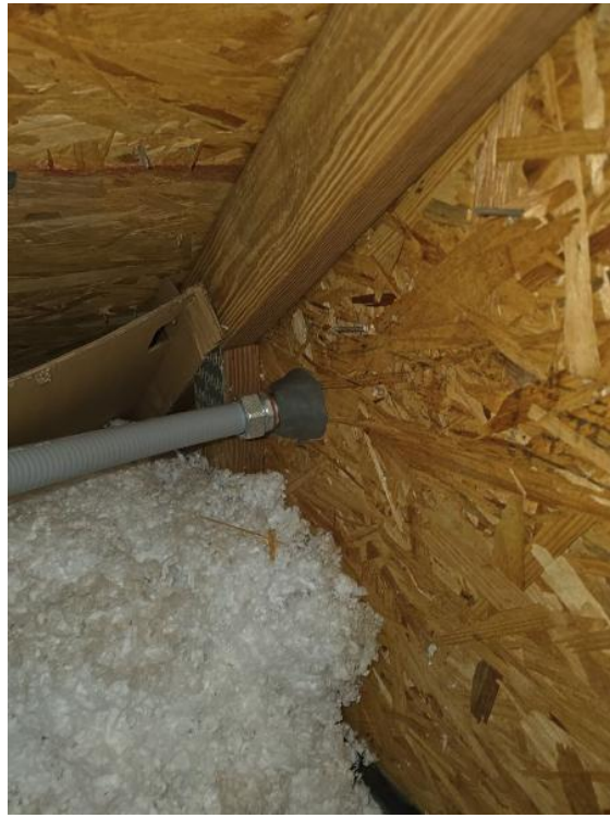
Attic / Sealed entry point
