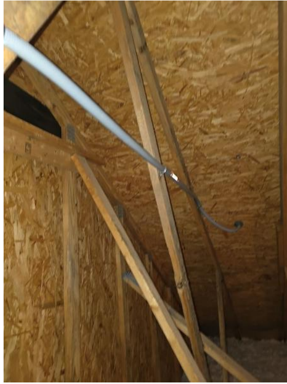
Attic / Attic conduit runs (3-4 images)
