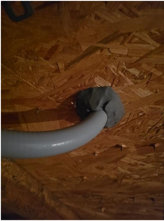
Attic / Sealed entry point
