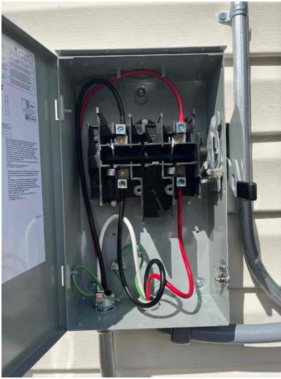
Electrical Equipment / Disconnect - With cover open
