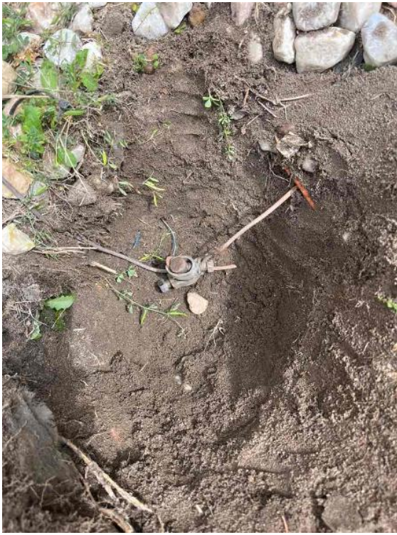
Electrical Equipment / Ground wire
